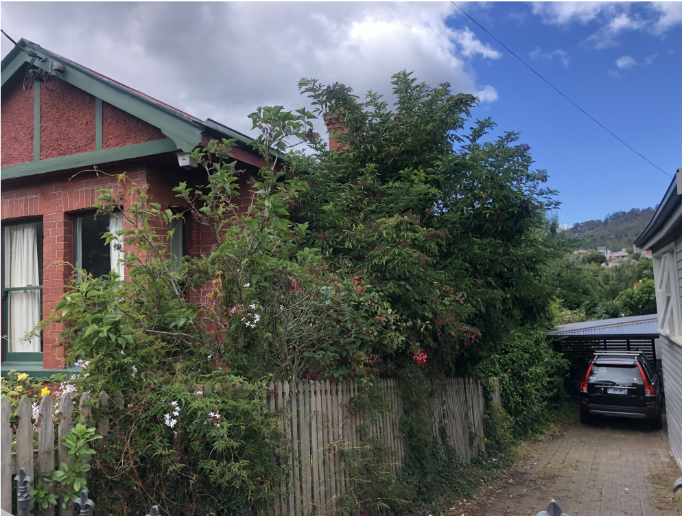
Figure 1. Photograph of the western elevation of 93 Princes Street. The dwelling and any views towards the proposed development are currently obscured by vegetation. If this was to be removed, it is likely that a narrow view corridor would exist. Source: Council Officer, January 2023.
