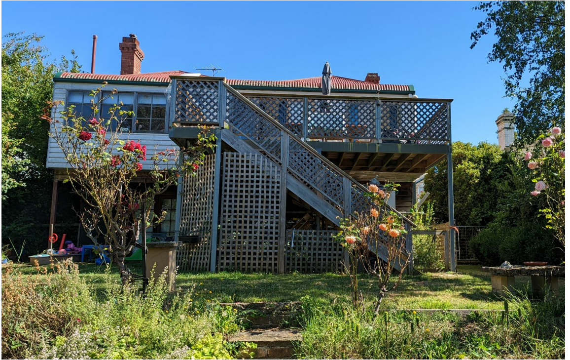
Figure 3: The existing rear elevation of the dwelling. Source: Officer photo.
