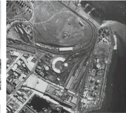
Figure 32: Aerial view of Mac Point, 1946
