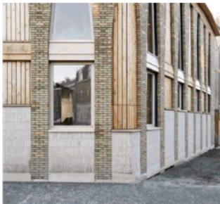
Figure 106: Boris Bouchet Architectes, Guillaume and Ramillien Architecture, 'Val de Scarpe' Education Center, 2019. Photograph Courtesy of Boris Bouchet.
