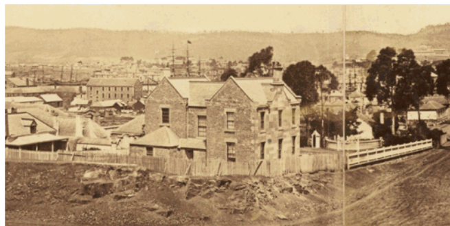
Figure 35: 1857 photograph showing the rear of the Royal Engineers Building, Hobart Town, from the Domain / Sharp photo., W L Crowther Library, State Library of Tasmania., SD_ILS:132002, AUTAS001136186327
