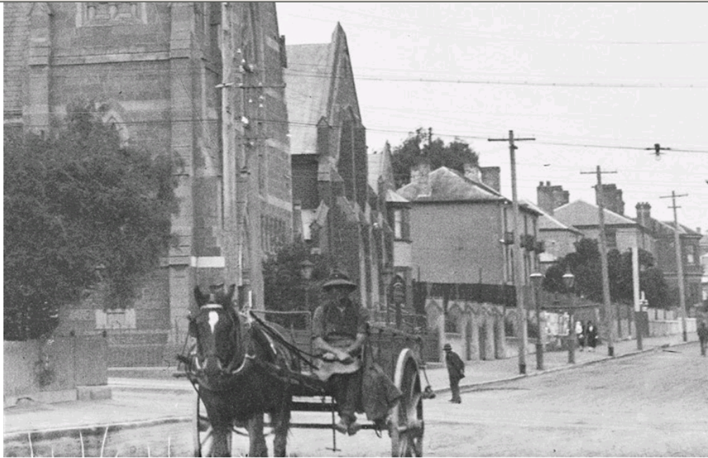
Figure 4.10 - C1915 Brisbane Street streetscape. TAHO NS1553-1-344
