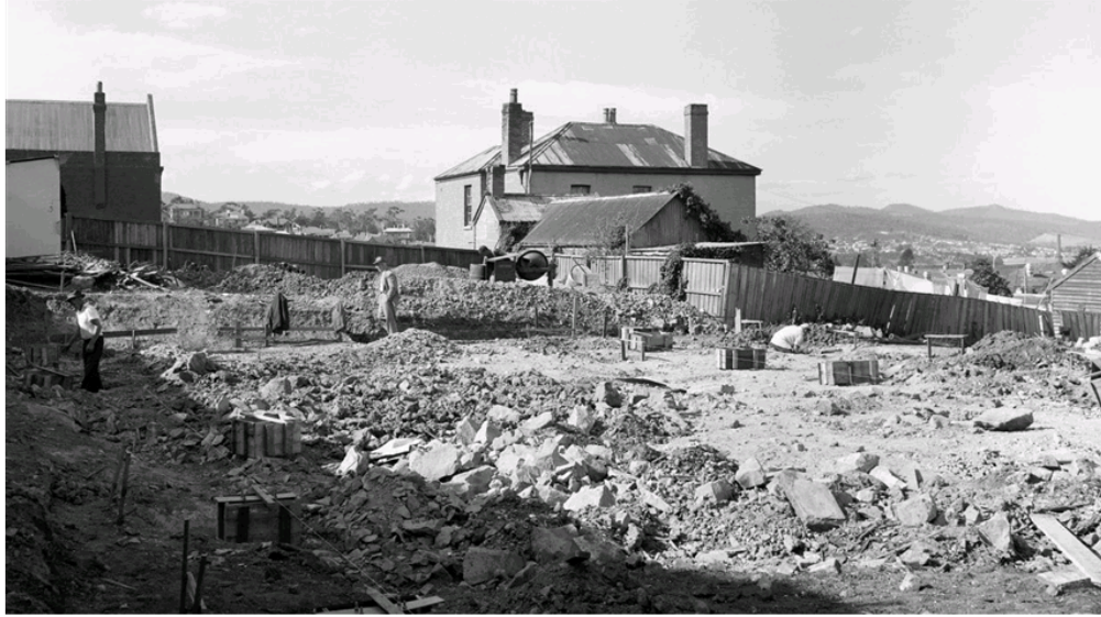
Figure 4.23 - Construction of the Teaching Aids Centre 1959. TAHO AB713-1-7048.
