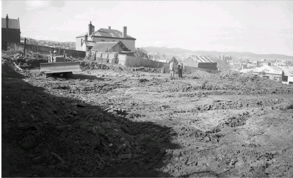
Figure 4.17 - Clearing for construction of the Teaching Aids Centre 1959. TAHO AB713-1-7041.
