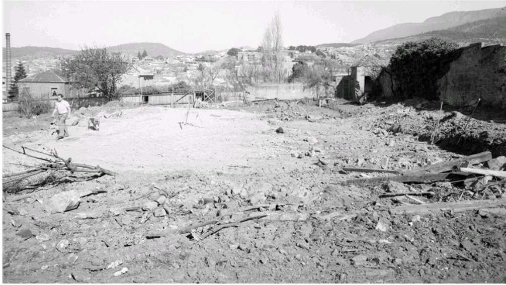
Figure 4.22 - Construction of the Teaching Aids Centre 1959. TAHO AB713-1-7043.
