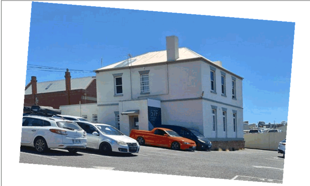
Photograph 5. Heritage building on site, formally Sydney Lodge.
