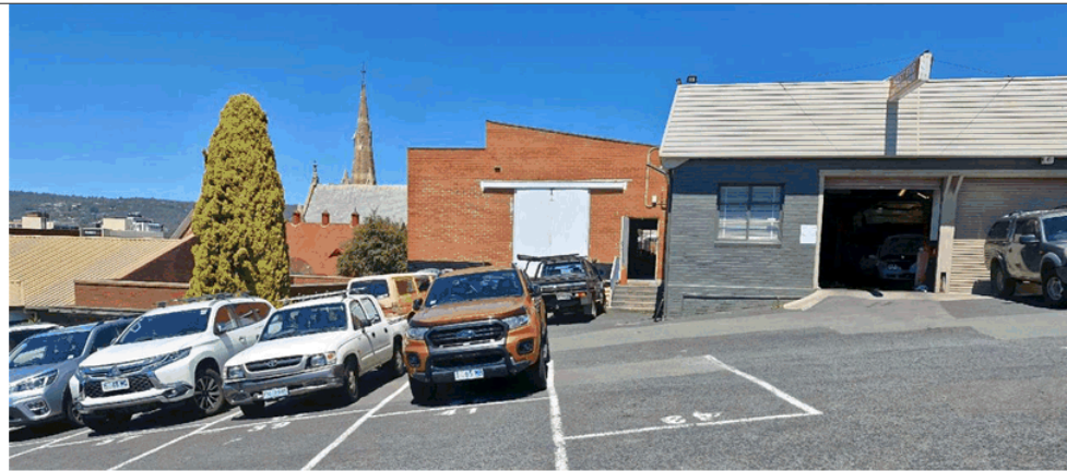
Photograph 6. Workshop and extension on site.
