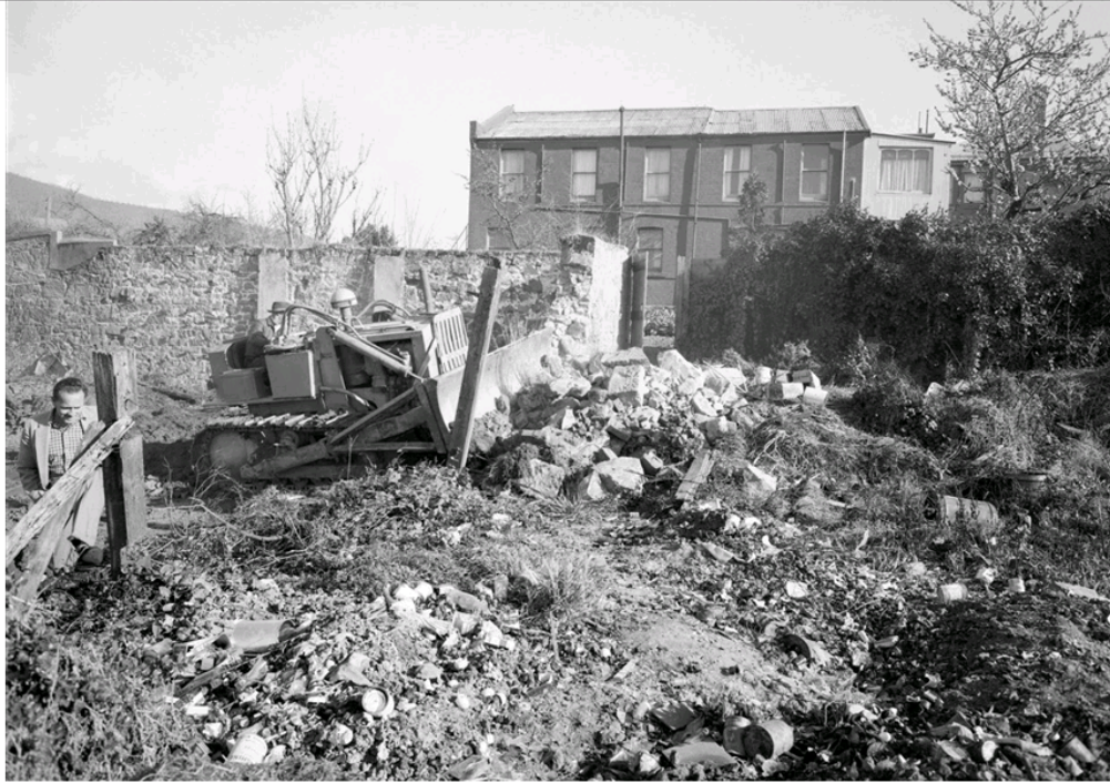
Figure 4.18 - Clearing for construction of the Teaching Aids Centre 1959. TAHO AB713-1-7036.
