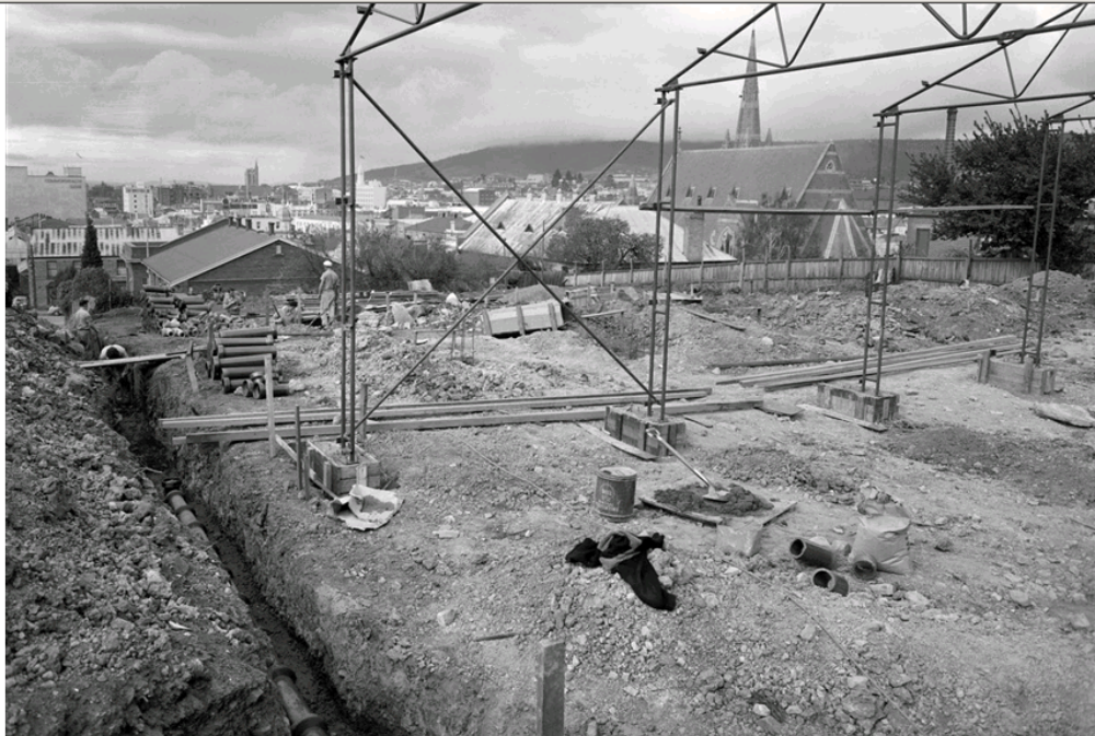
Figure 4.25 - Construction of the Teaching Aids Centre 1960. TAHO AB713-1-7098.
