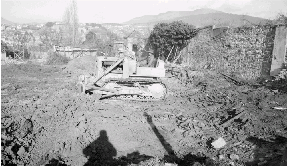
Figure 4.19 - Clearing for construction of the Teaching Aids Centre 1959. TAHO AB713-1-7037.
