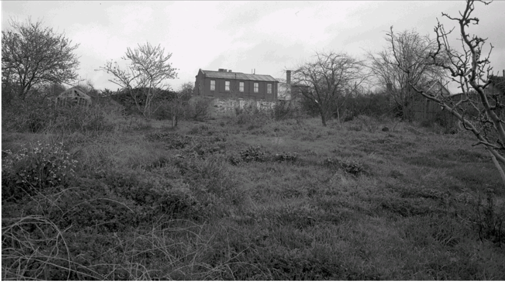
Figure 4.16 - Looking up the site prior to the construction of the Teaching Aids Centre 1959. TAHO AB713-1-7034
