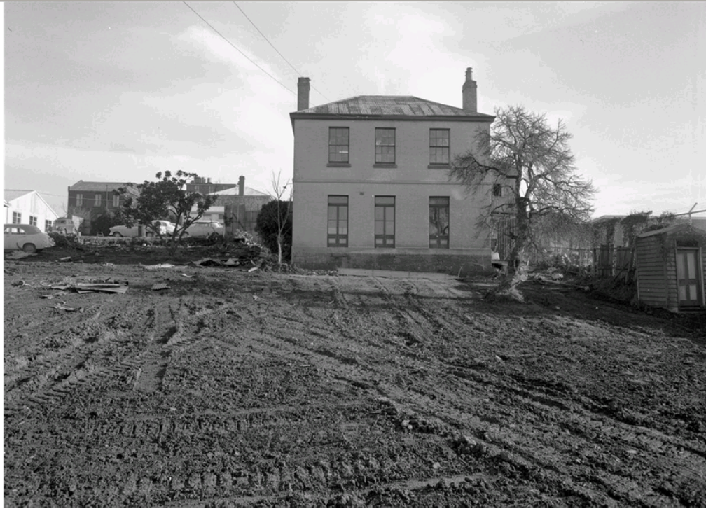
Note the earlier glazing arrangement of the building.
