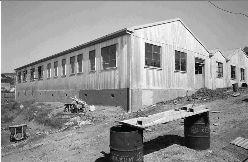
Figure 4.27 - Construction of the Teaching Aids Centre 1960. TAHO AB713-1-7158.
