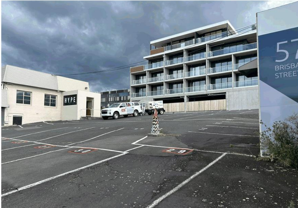
Figure 5.7 – Ingomar Apartments from the subject site.
