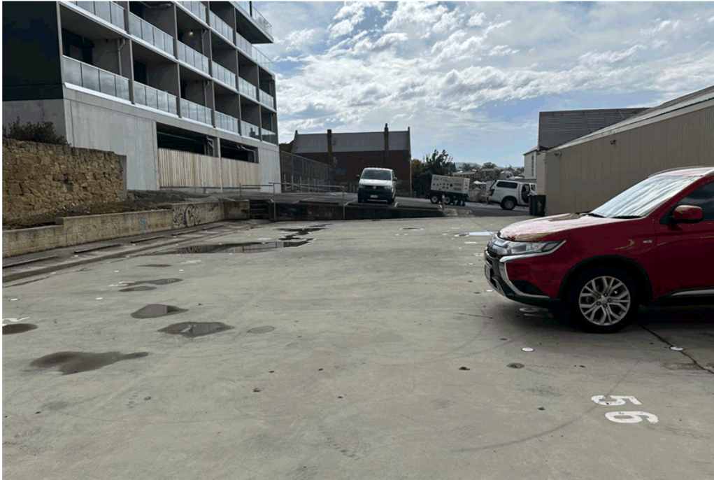
Figure 7.6 – Excavation at the rear of the site (top of the Hunt grant) to form a flat terrace for the northern bay of the Teaching Aids Building in 1960 – the slab from that building now used for parking.
