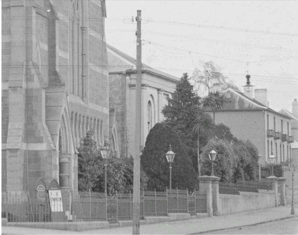
Figure 4.7 - C1900 Brisbane Street streetscape. TAHO NS392-1-752.
