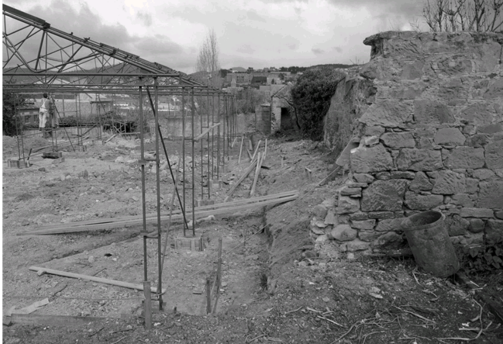
Figure 4.24 - Construction of the Teaching Aids Centre 1960. TAHO AB713-1-7011.
