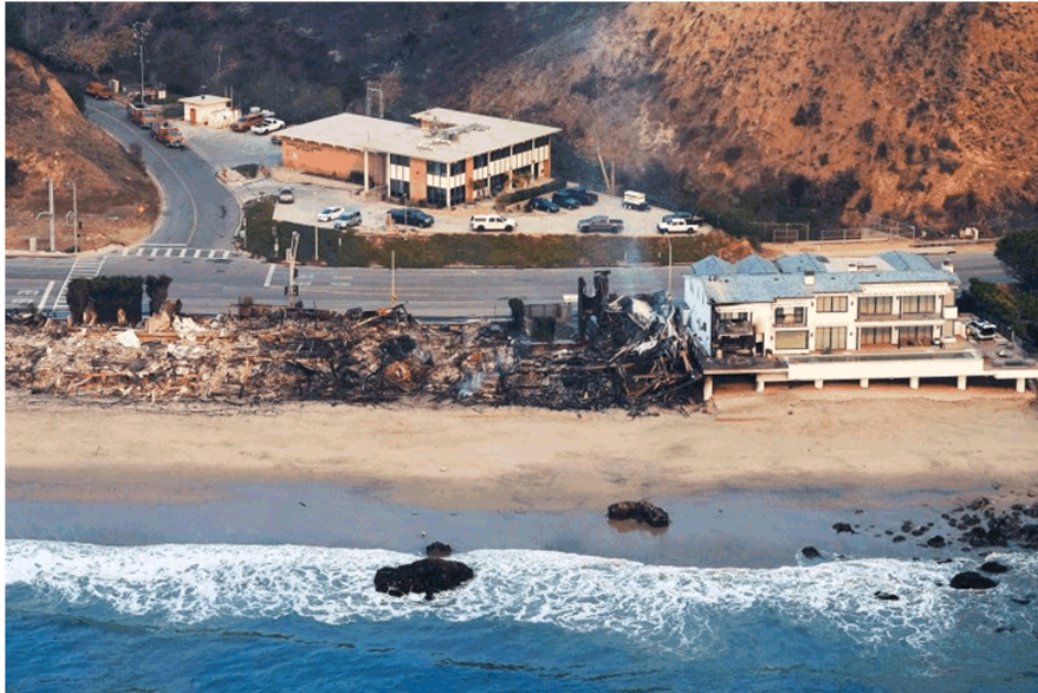
Figure 1: Beachfront properties destroyed by the Palisades Fire 4
