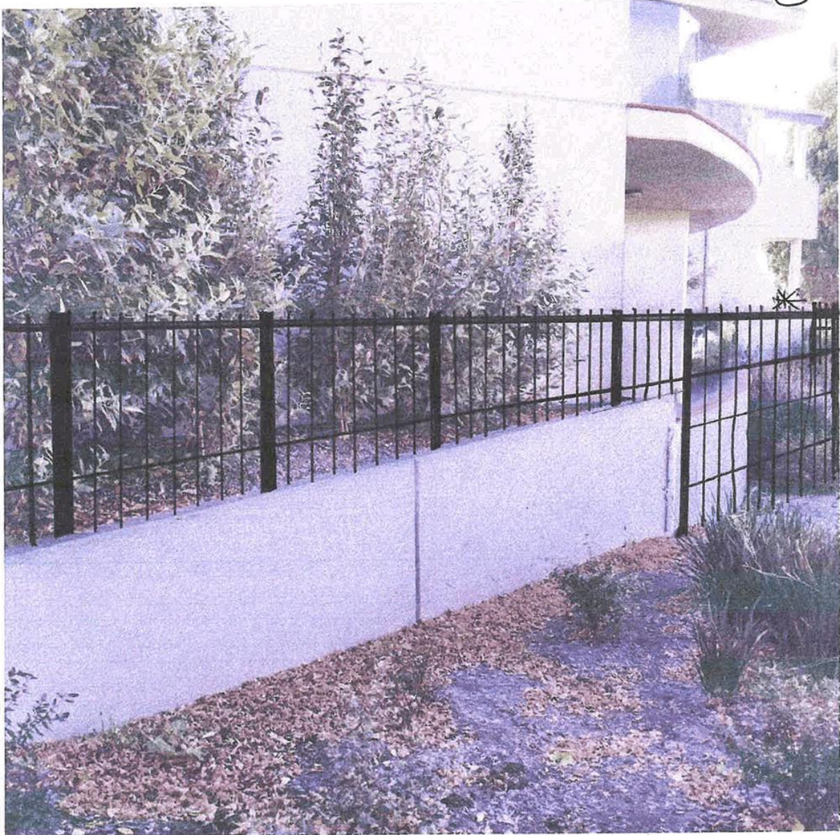
New full length fence continues on the boundary, then turns to attach to the wall of apartment 5. *
