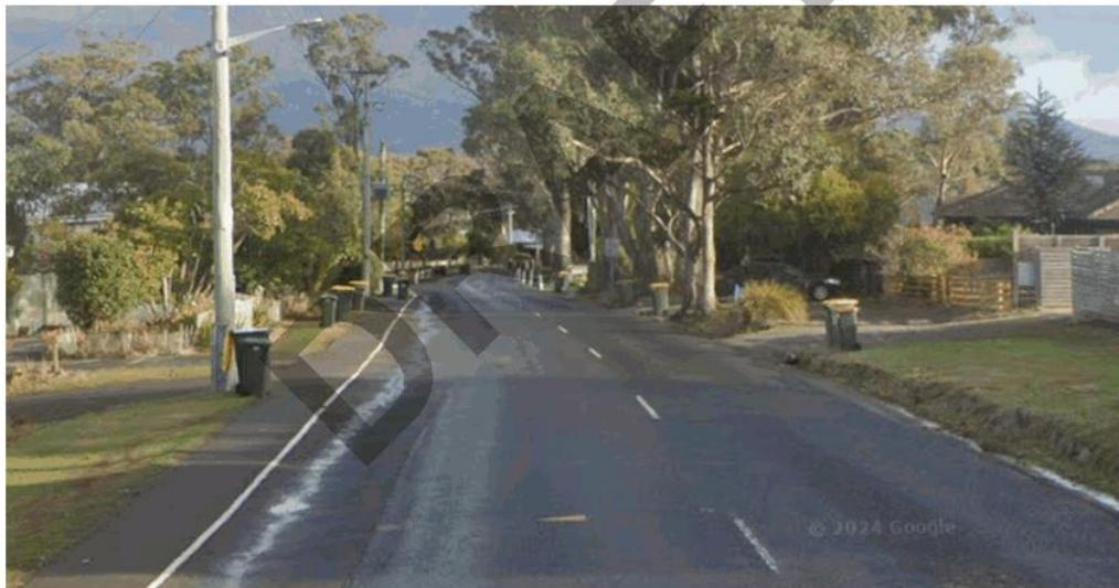
**Figure 3.10:** Nelson Road travelling west, where the lane width becomes excessive
