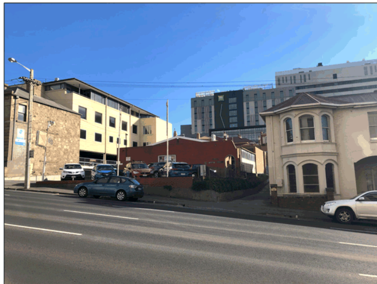
Figure 1 Views toward the subject site, currently occupied by a single storey face brick building of no heritage interest. Image taken July 2021.
