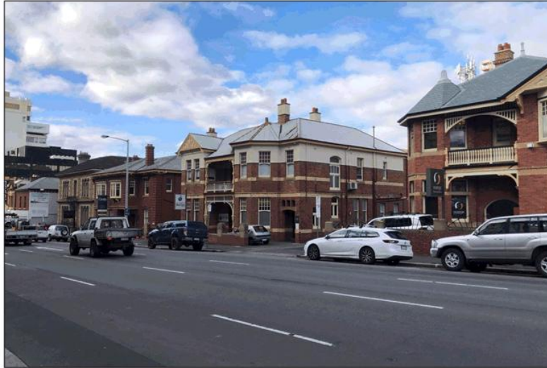
Figure 12 Southern side of Macquarie Street, looking north east. The building in the centre of the image, 176 Macquarie Street, is behind the subject site. Image taken July 2021.
