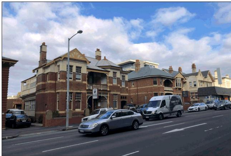
Figure 11 View of the heritage buildings along the southern side of Macquarie Street, adjacent to the rear of the subject site. The five storey envelope of the addition to the rear of 65-67 Davey Street is partially visible behind these structures. Image taken July 2021.
