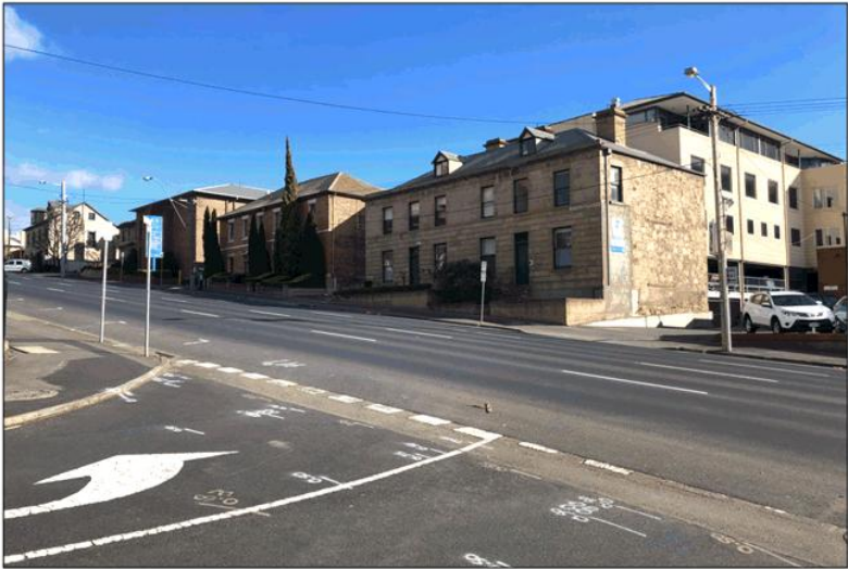
Figure 5 Northern side of Davey Street, facing south west with views toward the five storey addition to the rear of 65-67 Davey Street. Image taken July 2021.
