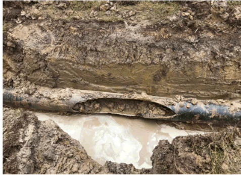
Figure 6.7. Typical condition of a water mains that require replacement
