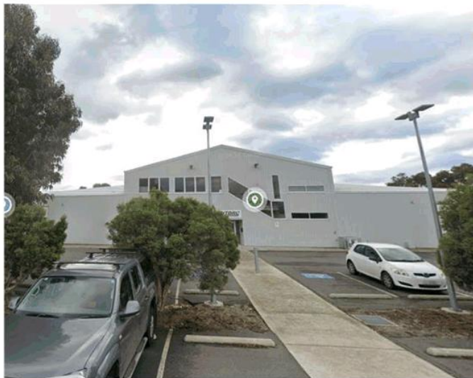
Figure 2: The New Town Bay Rowing Club building as seen from the car park. The function area is located within the upper storey.
