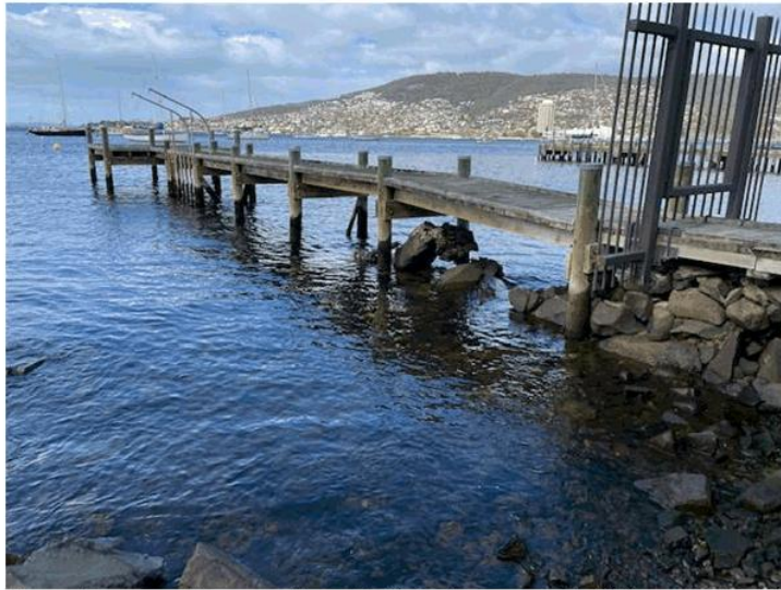
Figure 7: view of long section of jetty to be removed (Officer photo, 2025)
