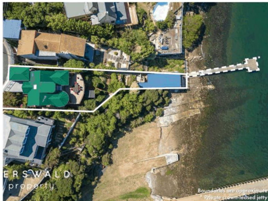
Figure 2: aerial view of previous boat slips in the vicinity of the subject site ( www.realestate.com.au , 2023)
