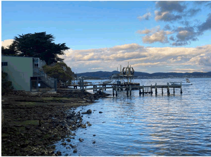
Figure 11: View of existing jetty from Perdon and Featherstone Reserve. Behind is another jetty structure which is currently under construction. (Officer photo, 2025)
