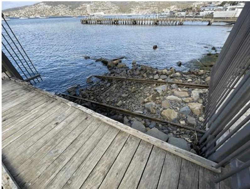
Figure 8: View of rails to be retained and rocks beyond to be location of new jetty (Officer photo, 2025)
