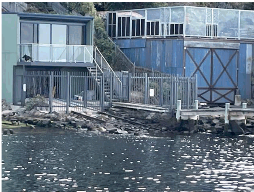
Figure 9: View of locaiton of new jetty to left of rails (Officer photo, 2025)
