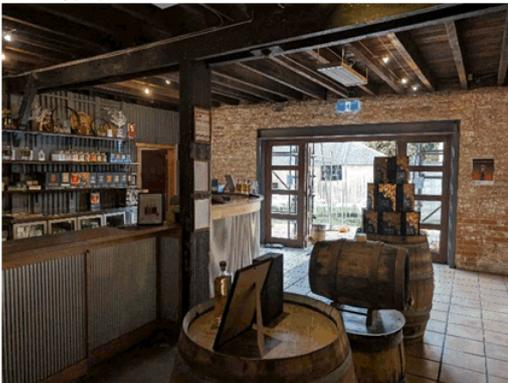
Figure 12: Ground floor bar with modern corrugated iron partition to be removed. Column to be retained.
