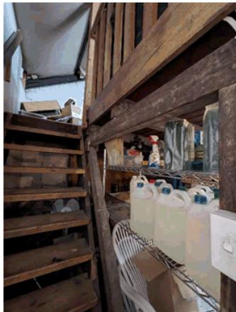
Figure 18: First floor view showing the bracing to be retained and modern balustrade above proposed for removal.
