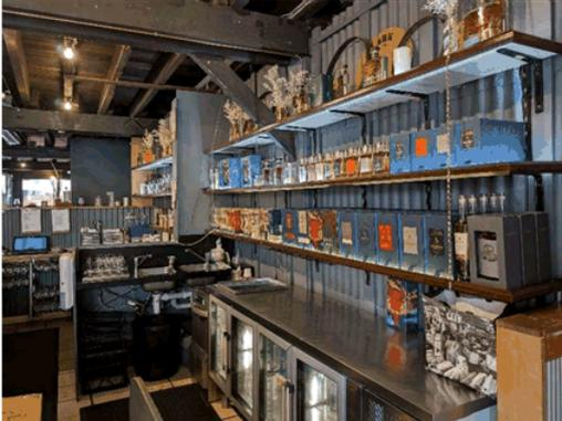
Figure 10: Ground floor bar with early / original corrugated iron partition to be retained. Wall beyond nib wall with modern corrugated iron lining proposed for removal.
