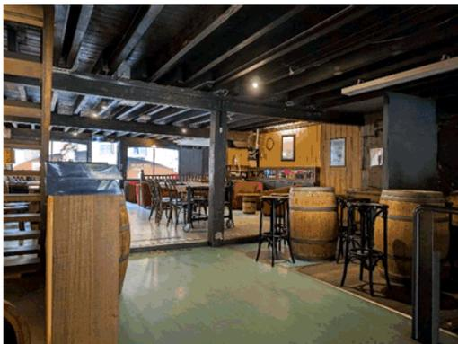
Figure 8: Ground floor raised floating floor and lino floor on top of original timber floorboards proposed for removal.
