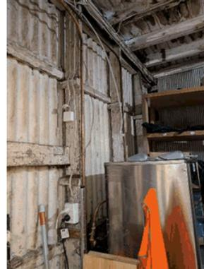
Figure 11: Ground floor back side of the early / original corrugated iron partition to be retained. Note profiled noggings.
