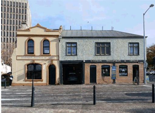
Figure 4: Northeastern (Argyle Street) elevation showing the battens projecting above the ridge that held signage.
