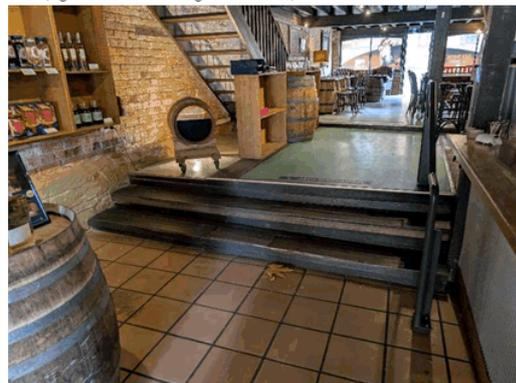
Figure 9: Ground floor modern steps proposed for removal and replacement with a platform lift and narrower stairs, timber stair to first floor beyond (left).
