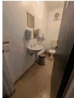
Figure 13: Ground floor toilet partitions, fixtures, and fittings proposed for removal, column in right side partition wall to be exposed and retained.
