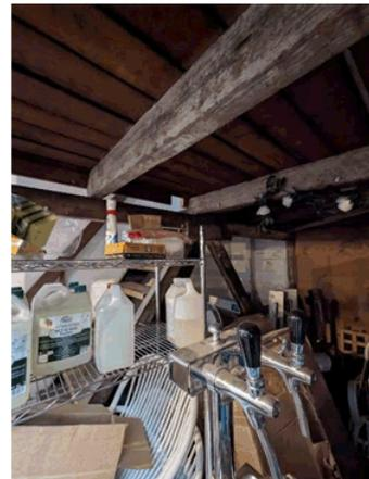
Figure 19: First floor loose-laid mezzanine floorboards to be removed and retained on site, joists to be raised to allow for a nominal clearance of 2100mm under.
