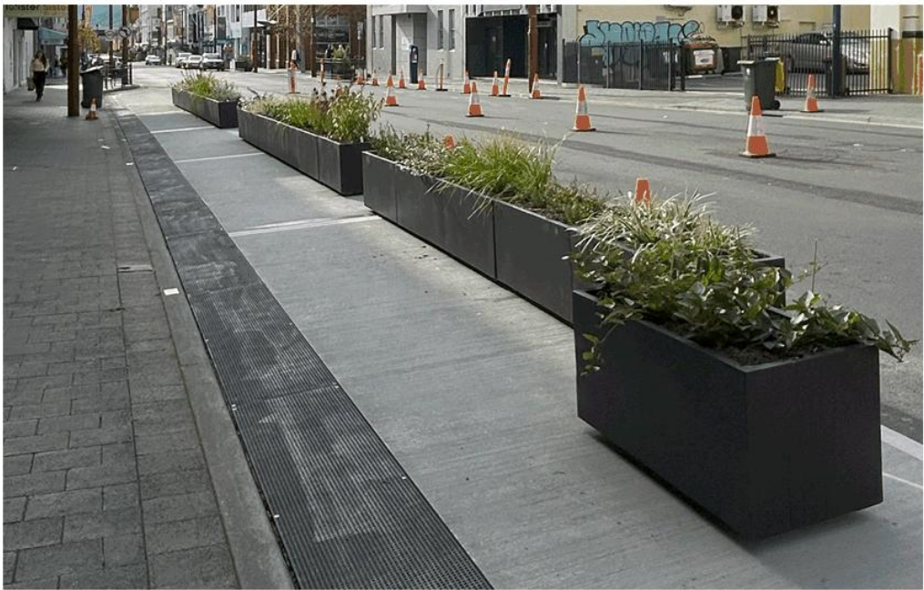
Figure 5. Typical footpath extension with concrete base and grating in Collins Street, planter boxes are optional and with additional cost.
