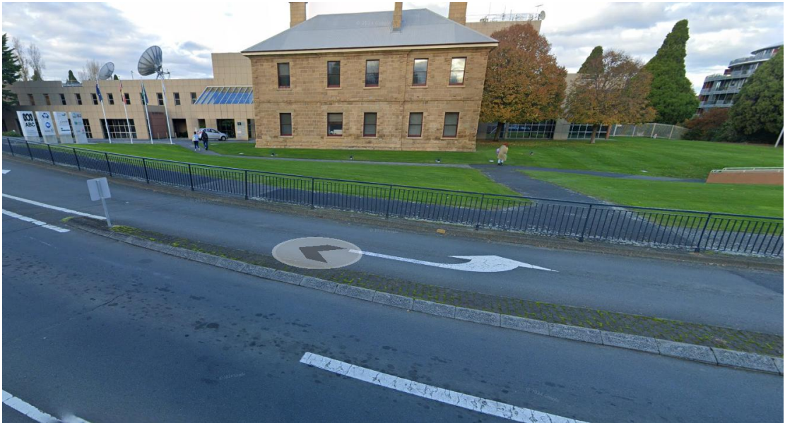
4.4. When fencing was installed as part of the construction of the railway roundabout the railway station was still in operation. At that time the
