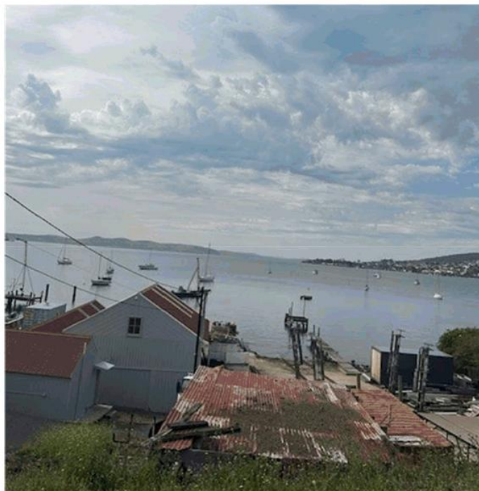
Fig. 3 – the subject site (Hunter's slip and associated outbuildings)– image taken by Council's Development Appraisal Planner
