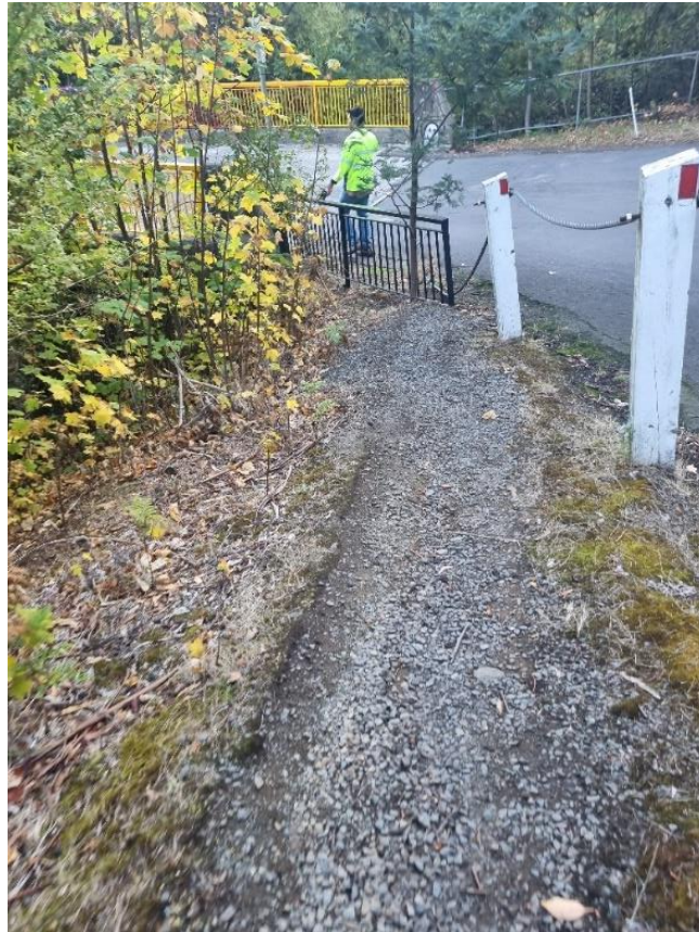
Photo 2 – Steep embankment on Romilly Street approaching Bridge looking southwest
