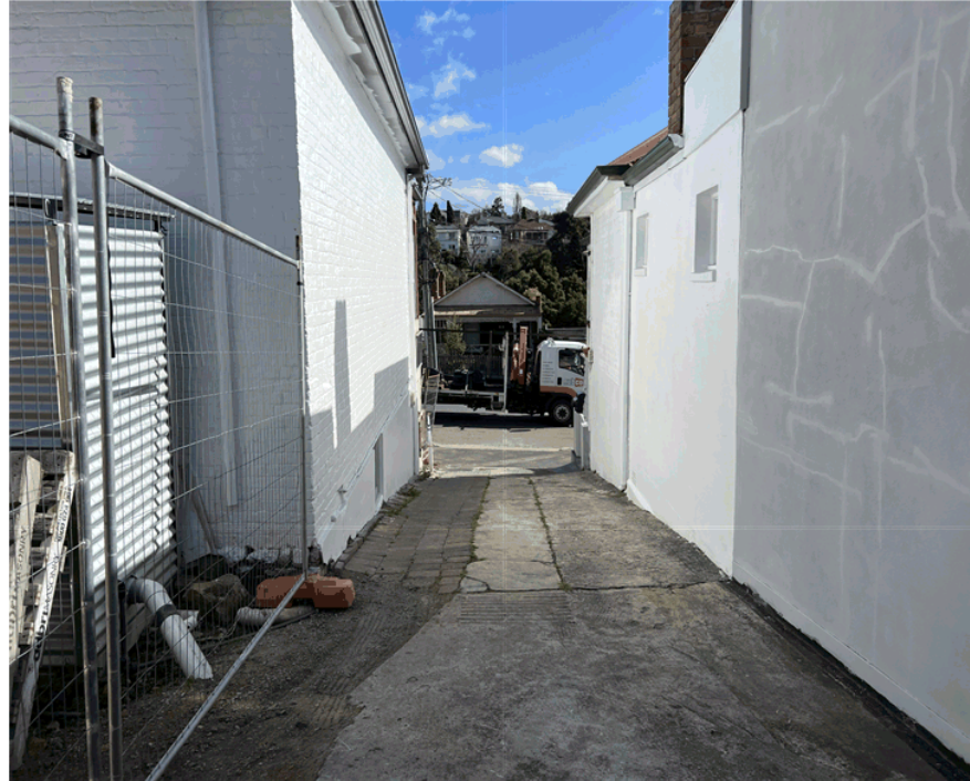
Figure 4: Sight Distances of access impeded. Note vehicles exiting the site would be doing so in reverse. (Officer Photo)
