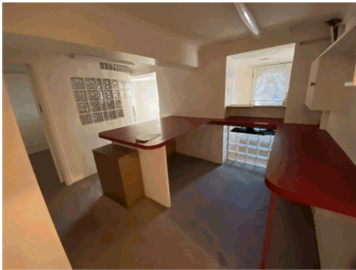
Figure 7: Existing block and glass wall
