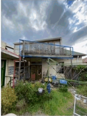
Figure 4: Existing deck to be removed
