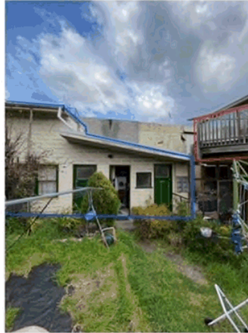
Figure 5: Outbuildings to be removed
