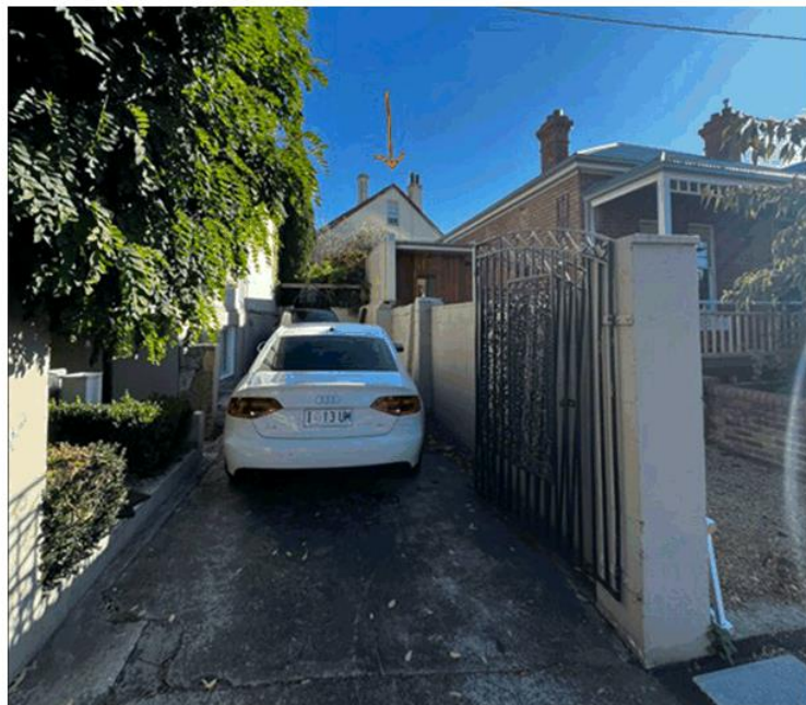
Fig 3. - 127 Warwick Street as viewed through neighbouring driveway (image taken by Heritage Officer April 2023)
