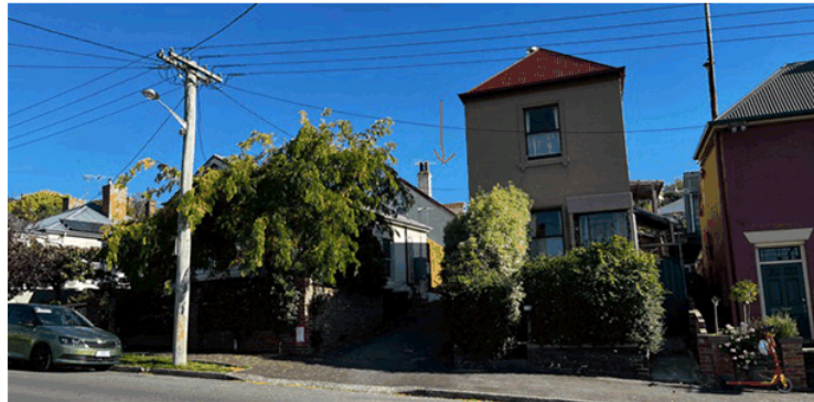
Fig. 1 - 127 Warwick Street as visible from Warwick Street, red arrow indicating property (image taken by Heritage Officer April 2023)
