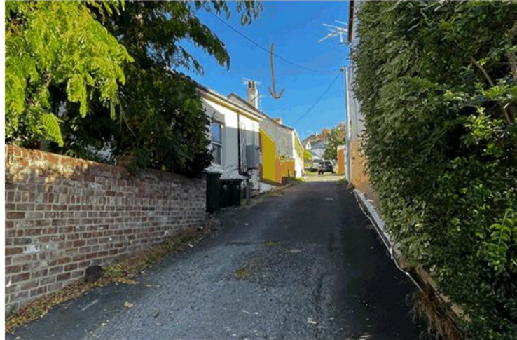
Fig. 2 - 127 Warwick Street as viewed from driveway, arrow indicating property (image taken by Heritage Officer April 2023)
