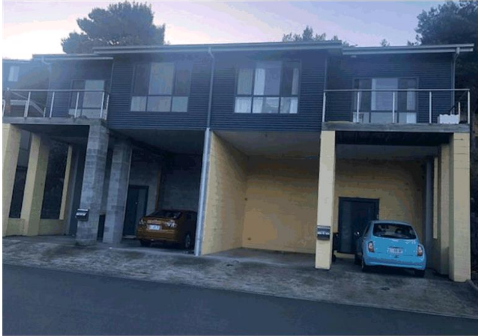
Fig. 7 - the subject site (on LHS) and 11/10 Waterworks Road
