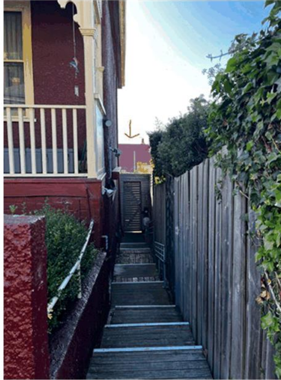
Fig. 4 127 Warwick Street as seen from Brown Street through gap in built form, arrow showing roof of property (image taken by Heritage Officer April 2023)
