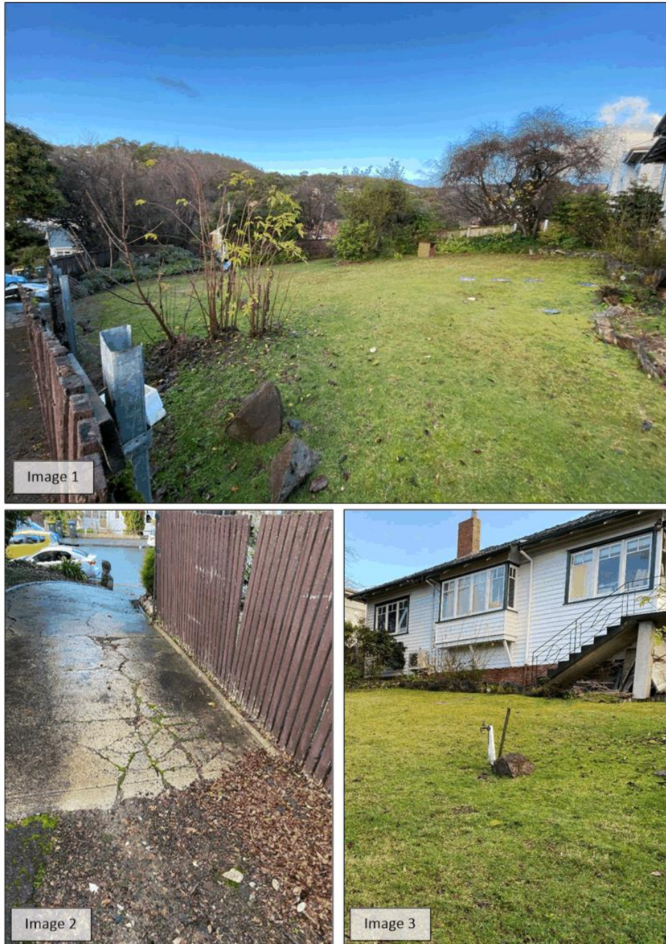
Figure 4: Image 1 = site surface with no signs of creep or slumping. Image 2 = cracked driveway concrete indicating highly reactive clays. Image 3 = the existing dwelling did not have major structural issues.
