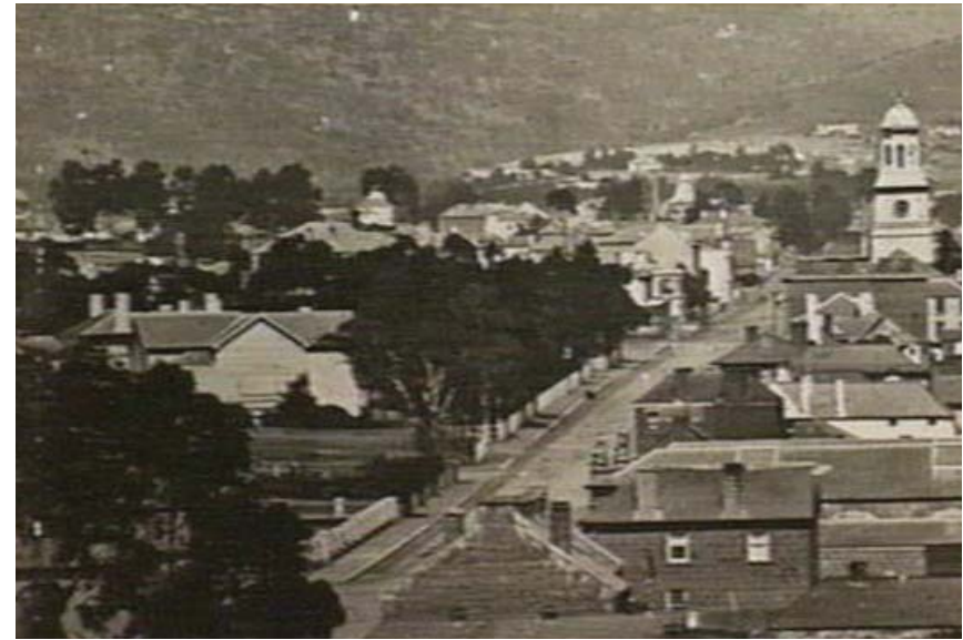
Fig 8 Macquarie Street frontage Photograph 1856, Portion of photograph Hobart: View from the Queens Domain, AC Dreier Collection, Latrobe Picture Collection, State Library of Victoria, H22002
