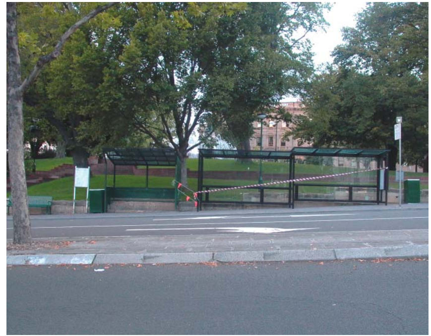
Fig 35 New bus shelters (in construction February 2007) have been used as an opportunity to recover some of the form of the sandstone base to the original cast iron fence.
