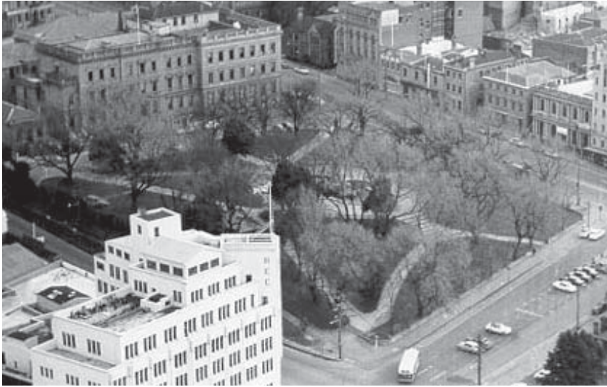
Fig 21 Aerial oblique view, shows asymmetrical layout and perrons on steeper slopes c. 1950 Archives Office of Tasmania 30/3099
