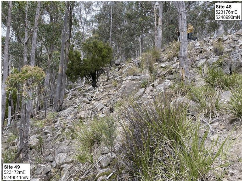
Plate 10. A view southeast and upslope towards Site 48 (top right), from near Site 49. The intervening rock-strewn slope is the outer face of a 35 – 40° spoil embankment from a sandstone quarry at top right. Boulder size ranges up to about 0.8 – 1m. The proposed track unavoidably crosses the lower part of the embankment at left of camera. It is suggested that some of the larger boulders be placed across the high side of the track to mitigate potential consequences of rock falls to track users.
