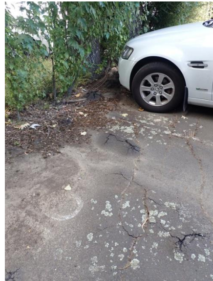
Figure 5. Large poplars 11 and 12 (far left) are damaging the car park surface – shallow roots of these trees are likely to impact / limit nearby structures.
