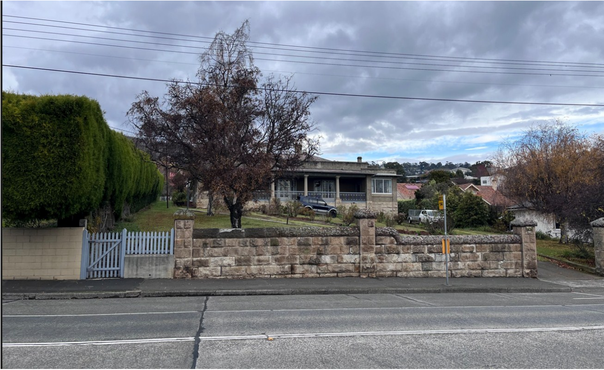
Subject site Preana 487 Sandy Bay Road (image taken by Heritage Officer)
