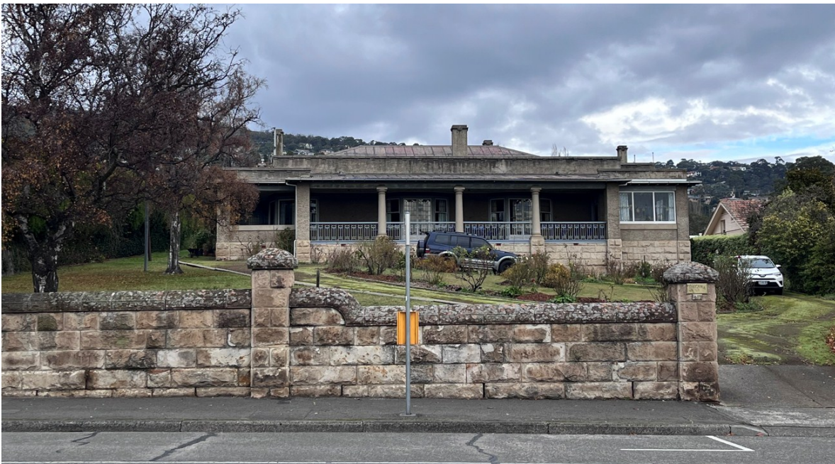
Subject site Preana 487 Sandy Bay Road (image taken by Heritage Officer)
