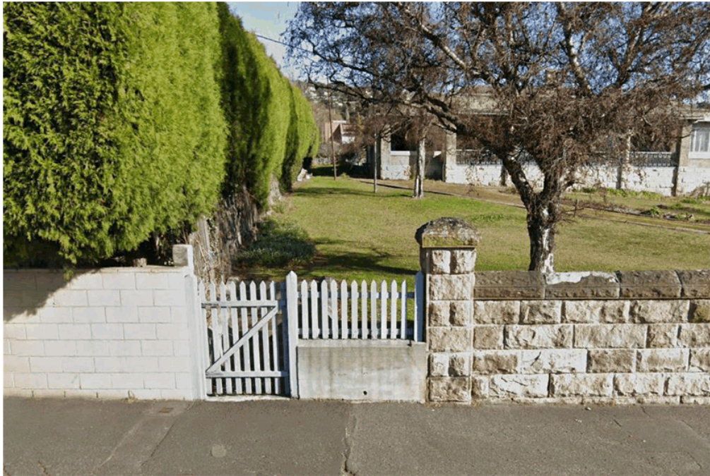
Existing legal access to the rear lot. Note that the picket fence is unlikely to be wide enough for compliant access, therefore the sandstone fence would require modification.
