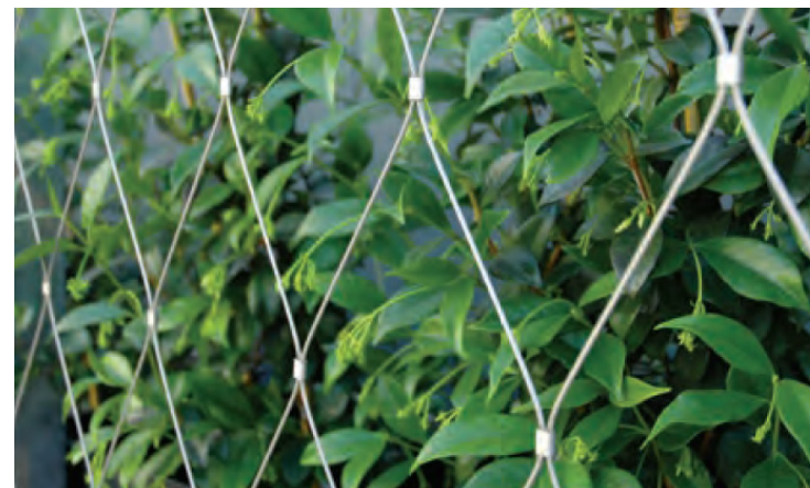
Stainless steel mesh - built example showing detailing
