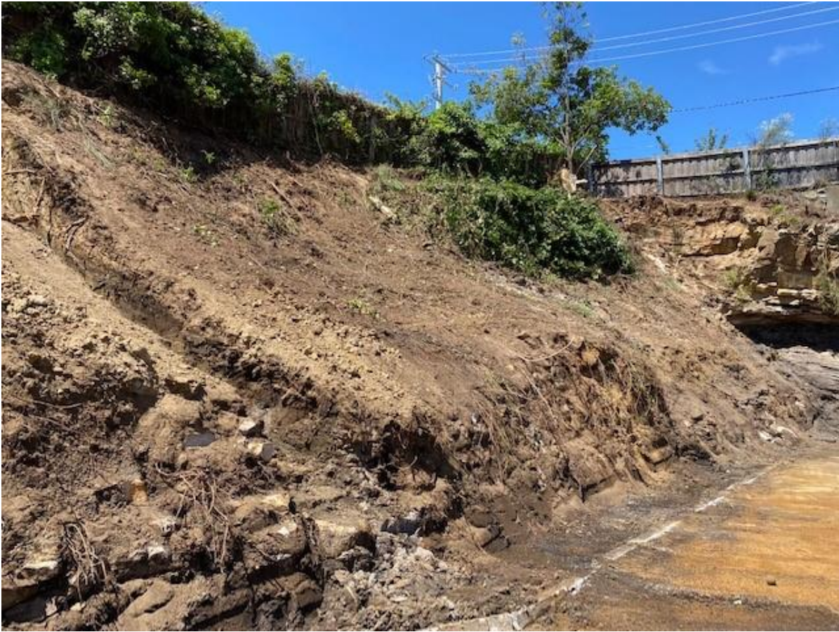
Figure 3. View of the north-eastern embankment with Trench 1 (LHS), showing sandy topsoil and sand/mudstone base. The sand/mudstone outcrop of the south-eastern wall is visible (RHS).
