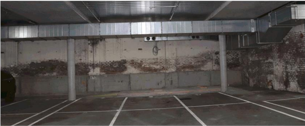
Figure 7.7 – Underpinned earlier wall in the basement carpark.
