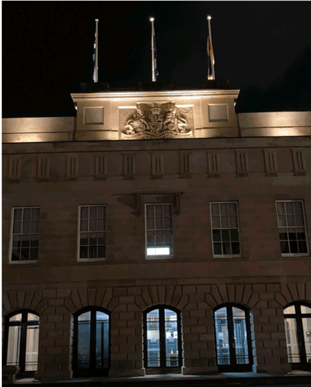
Parliament House lighting (PLN-20-150) using miniature spot lights for the flag poles and linear wall wash LED with stainless steel fastenings fixed into the mortar/grout. None of these are visible during the day.
