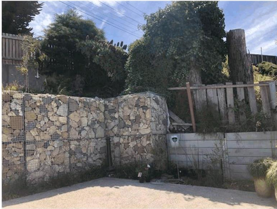
Existing wooden retaining walls on driveway not sufficient to accommodate additional traffic on premises and poses a risk to nieghbours and residents
