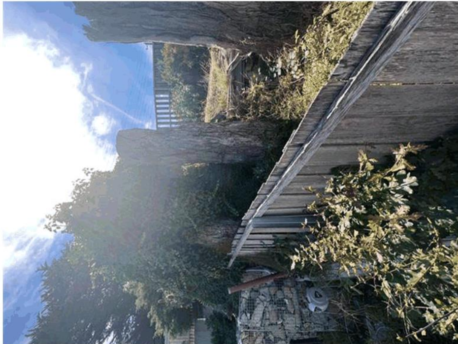
Existing wooden retaining walls on driveway not sufficient to accommodate additional traffic on premises and poses a risk to nieghbours and residents
