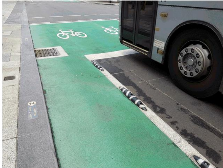
Figure 3.7: Protected 1.5 m feeder bicycle lane (Barrack Street, Perth) using Zicla Zebra separators
