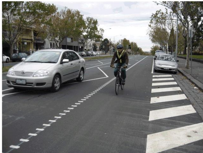
Figure 3.8: Audio-tactile line marking (Rathdowne Street, Carlton, Melbourne)
