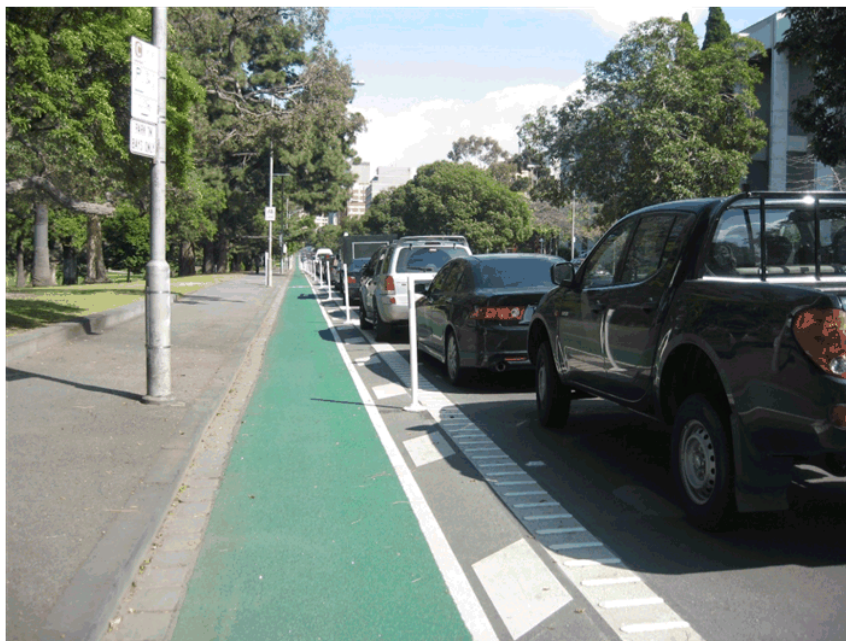
Figure 3.1: Albert Street (East Melbourne) - bicycle lane is 1.4 m wide and buffer is 0.8 m wide)
