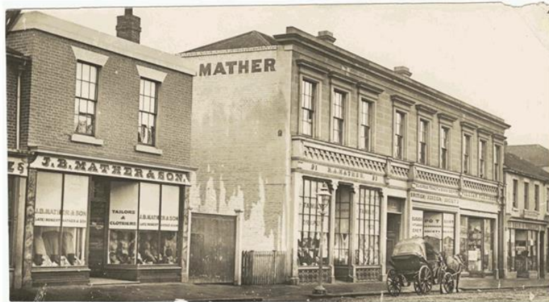
Photograph 1: Mather's Building at 91 Liverpool Street, c. 1880 (PH30/1/3997 Libraries Tasmania). Note that the brick side wall was limewashed, and the decorative frieze over the small pane shopfront windows. The fine detail of the frieze was lost when the present awning was constructed in 1919.
