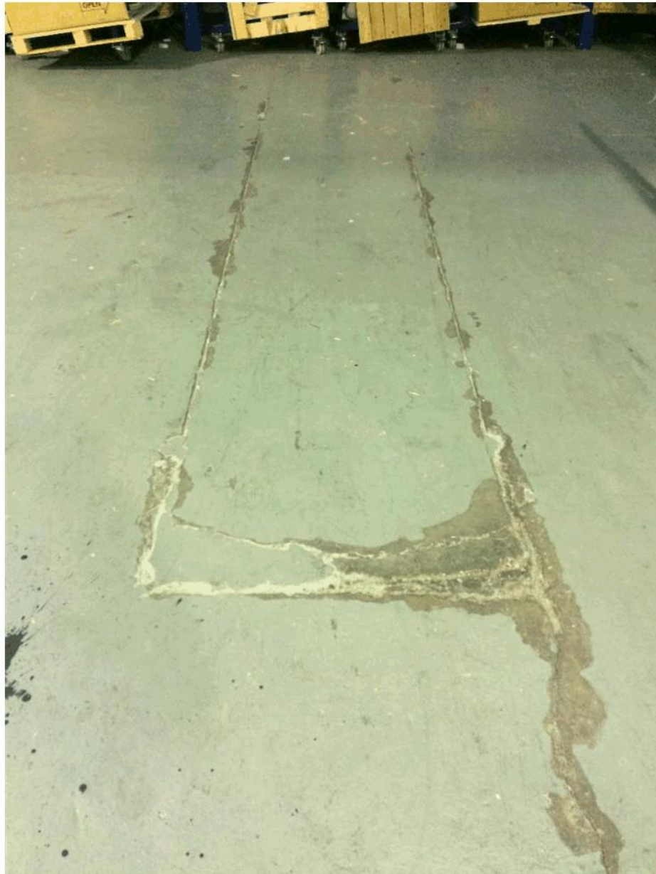
Plate 3 Rectangular section of flooring towards back of warehouse that may indicate replaced infrastructure or flooring
