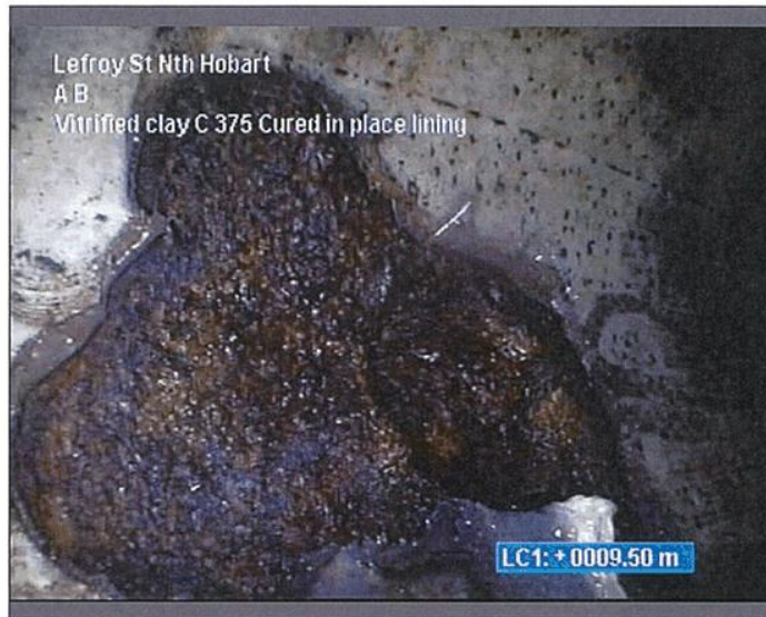
Photo: 1_1_4_A.JPG, Media No.: 300517_1, 00:03:12 9.5m, The re-establishment of a connection has been done improperly, reduction in cross sectional area: 5-20%, poorly cut open (to large), at 10 o'clock
