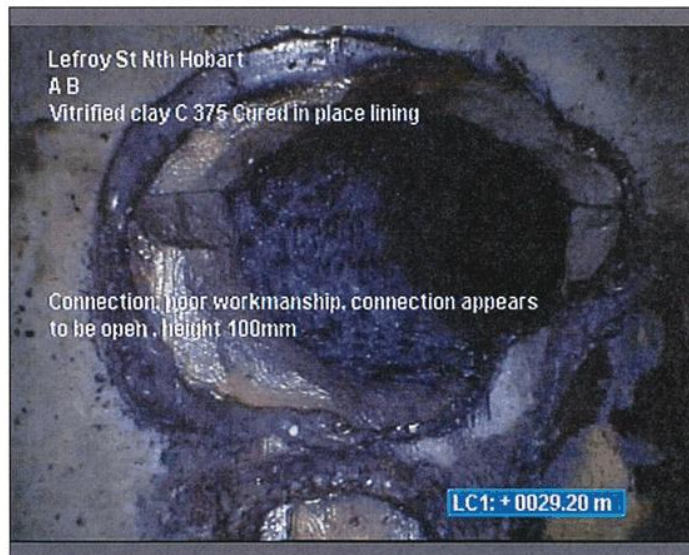
Photo: 1_1_6_A.JPG, Media No.: 300517_1, 00:07:34 29.2m, Connection, poor workmanship, connection appears to be open , height 100mm
