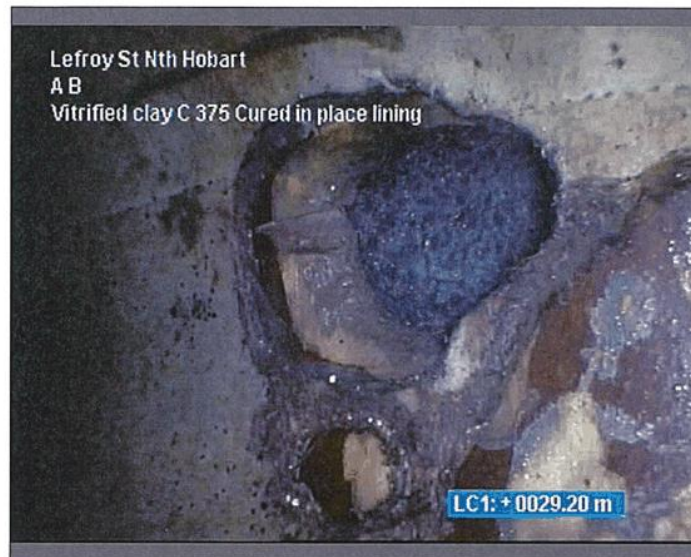
Photo: 1_1_6_B.JPG, Media No.: 300517_1, 00:07:34 29.2m, Connection, poor workmanship, connection appears to be open , height 100mm
