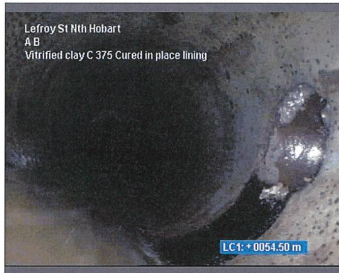
Photo: 1_1_8_B.JPG, Media No.: 300517_1, 00:11:46 54.5m, Junction open, good workmanship, height 100mm , at 2 o'clock
