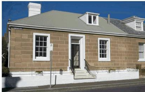
Subject property without signage in 2007. Source: Council image
