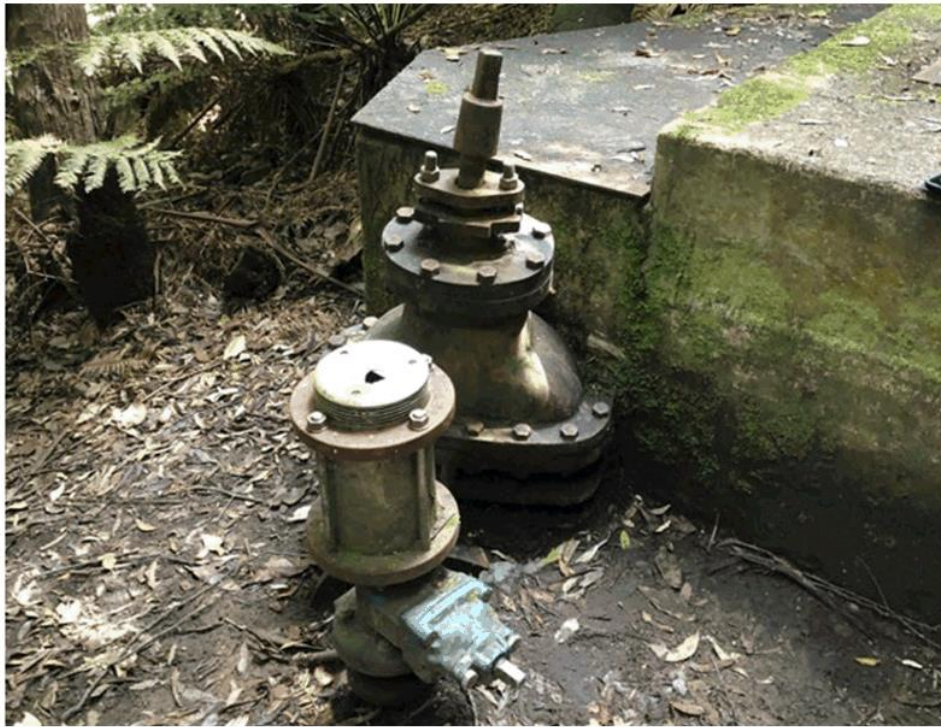
Figure 6: Existing manual valve
