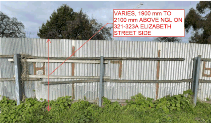
IMAGE 2: TYPICAL CONSTRUCTION DETAIL OF EXISTING BOUNDARY FENCE
