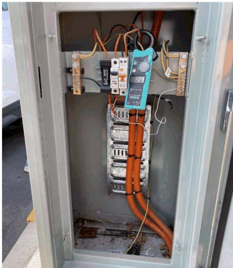
Figure 2: Lefroy Street entrance switchboard (ammeter reading shown with 6 of 10 lights turned on)
