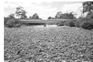
The number of piers and footings should be kept to a minimum in stream channels
