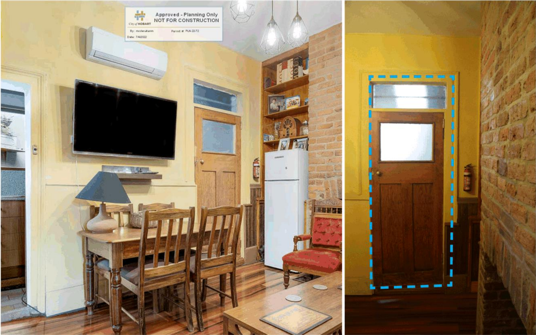
#12 - REMOVE EXISTING BATHROOM DOORWAY & WINDOW OVER
