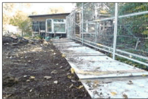
Ground protection image 1: Heavy-duty plywood set onto a compressible woodchip layer and pinned into position is suitable to spread the loading from pedestrian access.
