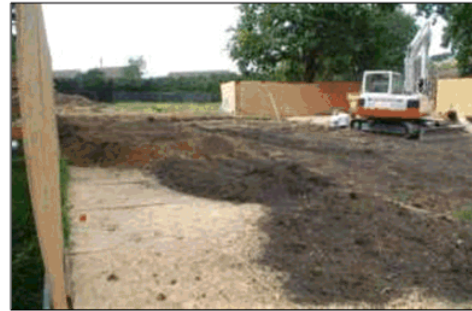
Ground protection image 2: Spreading soil excavated from footings is an effective way of buffering the plywood surface from the wear of light vehicles.
