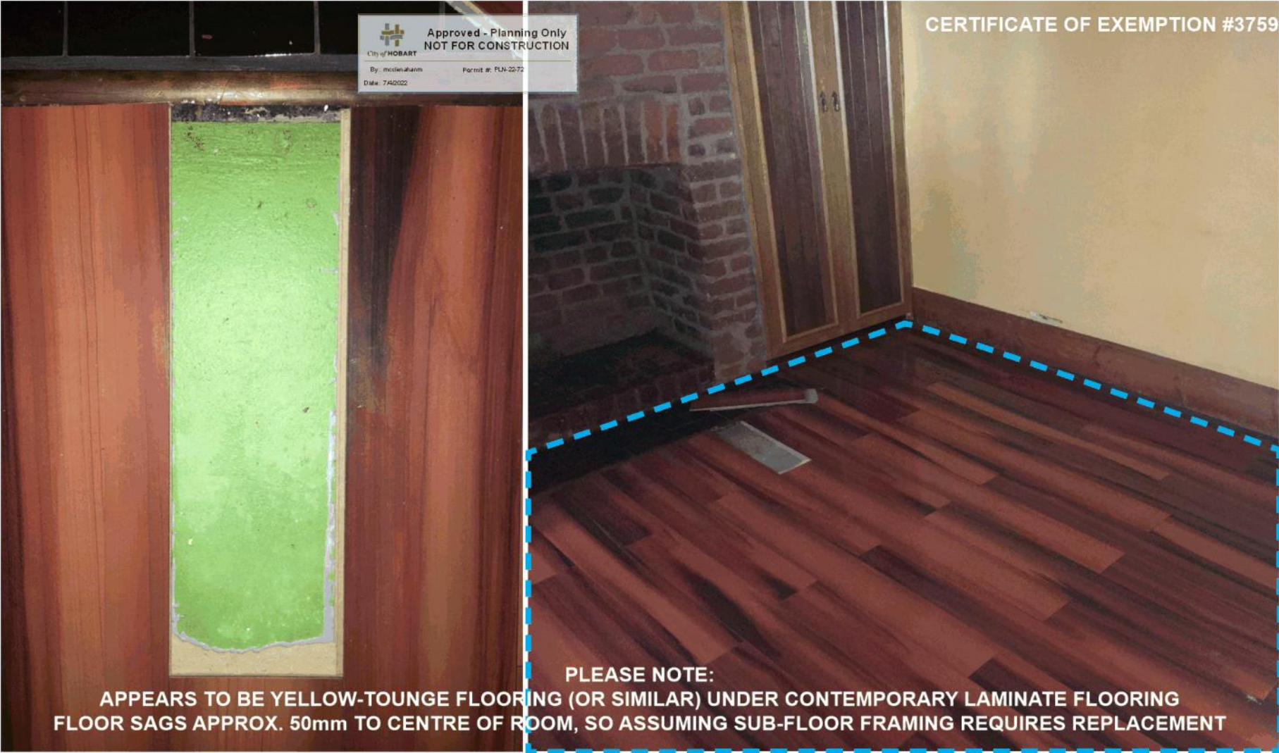
#10 - REMOVE CONTEMPORARY LAMINATE FLOOR COVERING, YELLOW TONGUE FLOOR UNDER & SUB-FLOOR FRAMING
