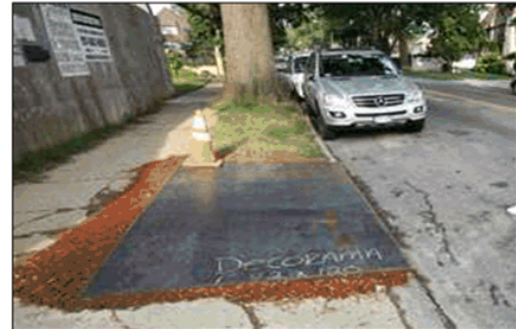
Ground protection image 8: Steel plates can be an effective way of temporarily reinforcing weak surfacing over a construction access during the development activity.
