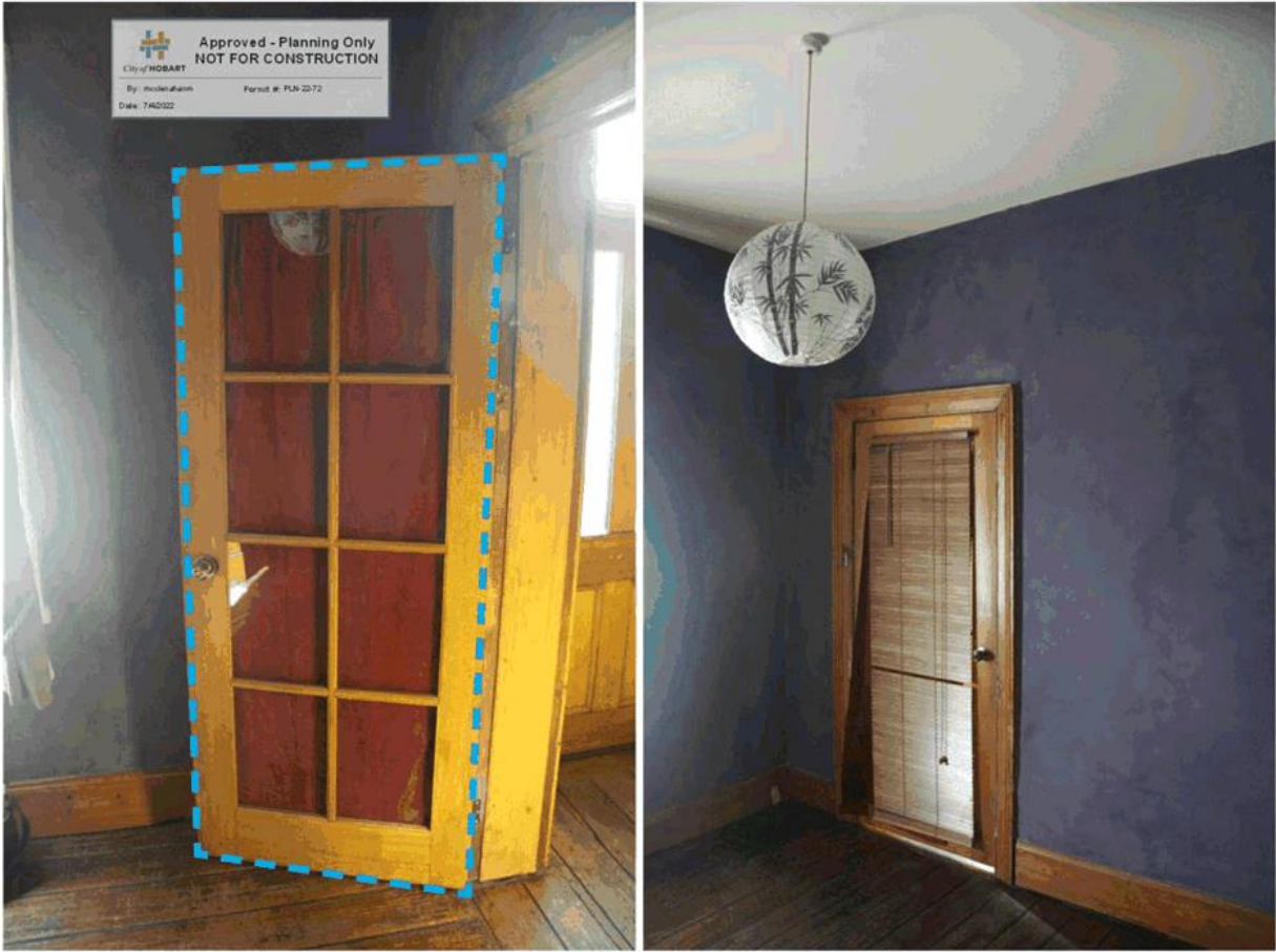
#15 - REMOVE CONTEMPORARY DOOR, RETAIN ARCHITRAVE
