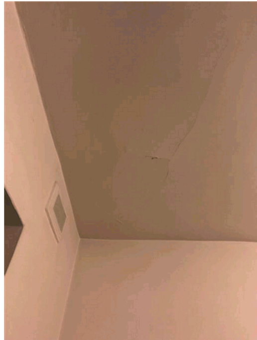
Water leaking through ceiling in bedroom
