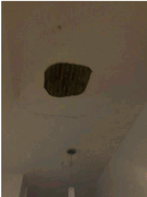
Lath and plaster ceiling collapse in hallway
