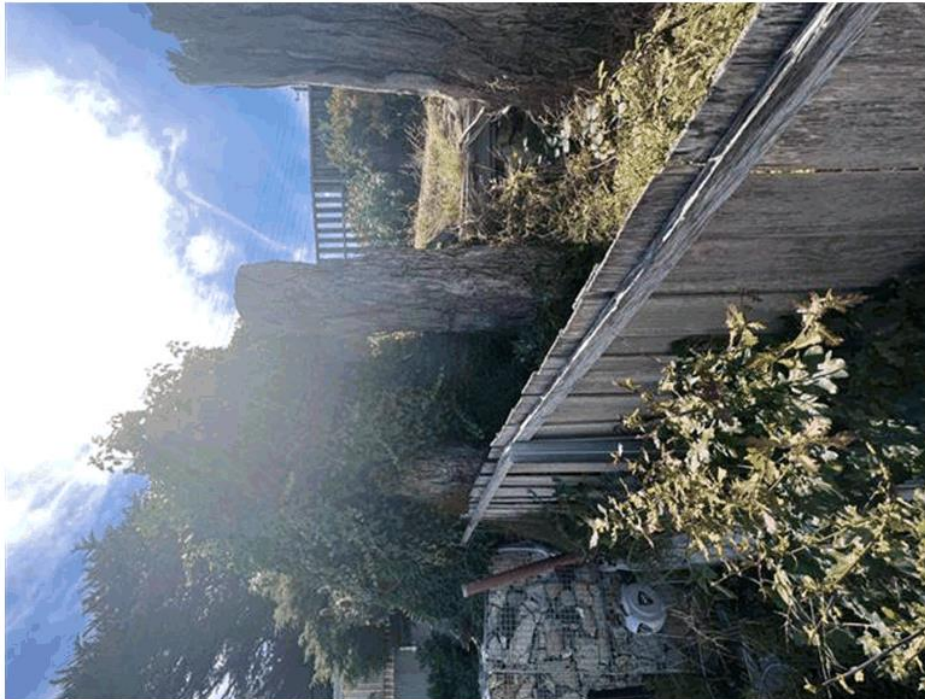
Existing wooden retaining walls on driveway not sufficient to accommodate additional traffic on premises and poses a risk to neighbours and residents
