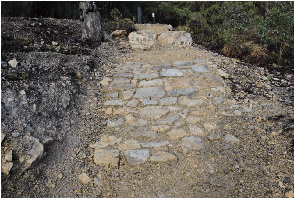
Rock armoured landing zone prevents erosion
