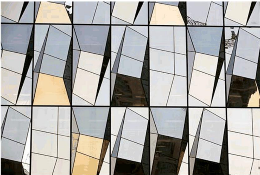
Figure 37 – facade detail of the Trutec Tower in Seoul, designed by Barkow Leibinger Architects and showing the effect of subtle re-orientation of facade glazing to achieve fractured reflectivity
