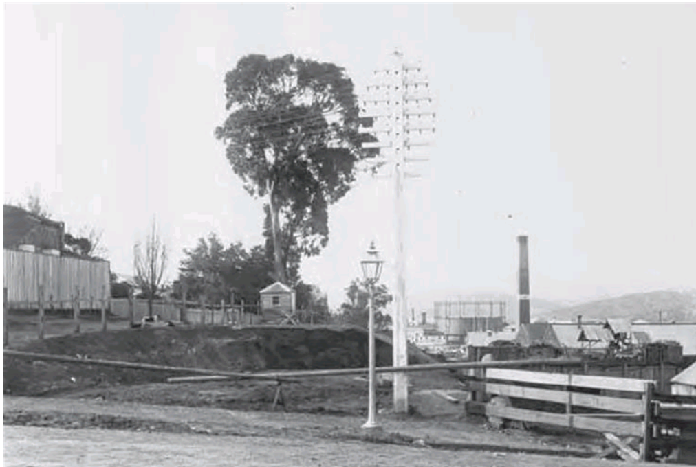
Figure 3.2.16 - Looking up Davey Street, c1890. This image appears to show the commencement of the widening of Davey Street, with excavation of the remnants of the escarpment for the lower level of the street. Note the Risby buildings to the right of the photograph, showing a range of timber sheds. Tasmanian Museum and Art Gallery (Q6411 HCC1890/82)
