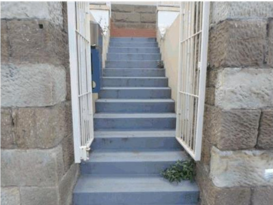
Plate 10: The main entrance through the stone wall feature showing the original sandstone pillars on the wall entrance and the later addition of the concrete stairs
