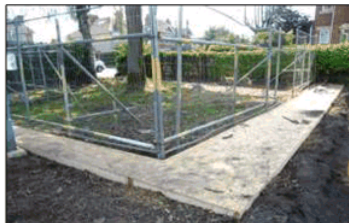
Ground protection image 3: Plywood fixed to a wood frame is another effective method of protecting soil from pedestrian compaction.
