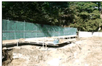
Ground protection image 4: A scaffold framework attached to the main scaffold fencing can be used to support either scaffold planks or plywood to create an elevated platform with a gap beneath.
