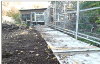
Ground protection image 1: Heavy-duty plywood set onto a compressible woodchip layer and pinned into position is suitable to spread the loading from pedestrian access.
