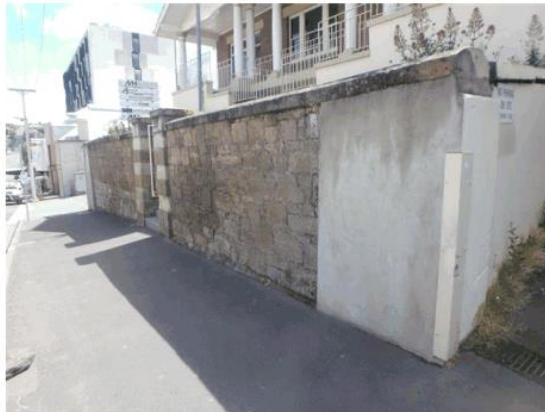
Plate 8: The section of the wall demolished during the 1960s for the widening of the driveway and the concrete section of replacement
