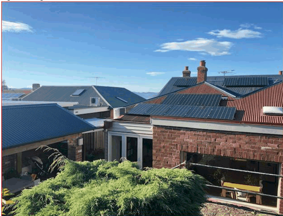
Fig. 9 .existing rear elevation - the roofed open sided building to the left of the photo and the white weatherboard and brick sections will be demolished to allow the proposed extension to be constructed. The peaked section of the roof will be retained.
