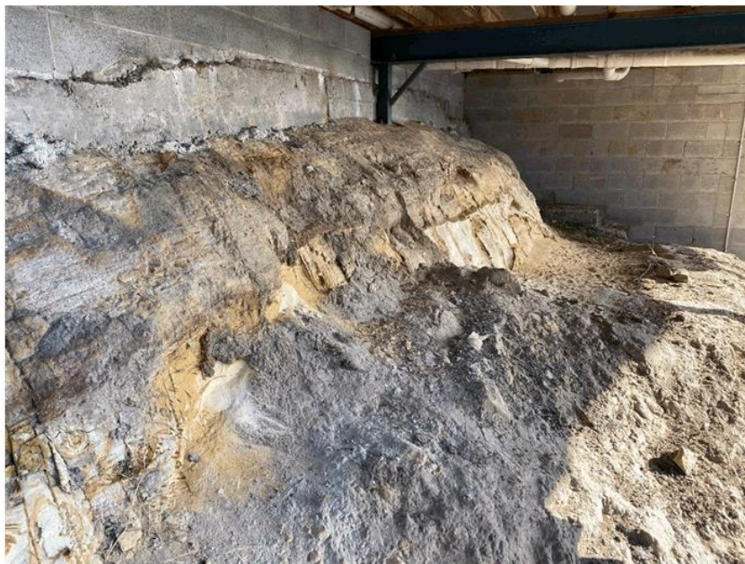
Figure 3: Cutting under neighbouring property showing competent Triassic sandstone bedrock. Cutting is at similar slope elevation to proposed site.
