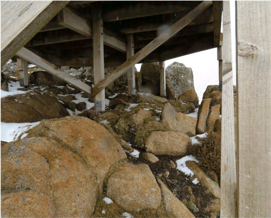
Photo 6 - Viewing platform construction on dolerite outcrop
