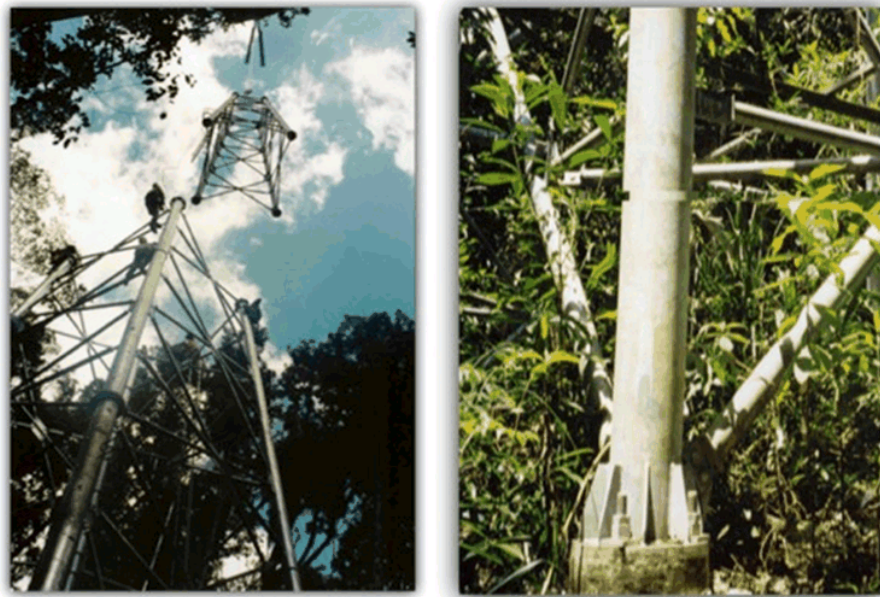
Figure 3 Tower components installed by helicopter, with vegetation regrowth following construction. Source: (Vos, 2018)
