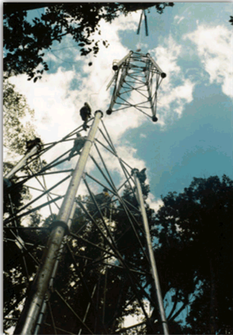
Figure 2 - Tower components installed by helicopter
