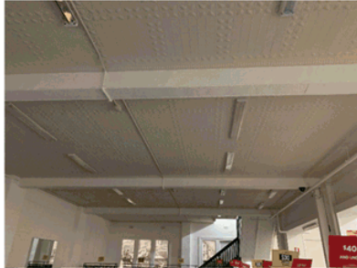
Figure 17 - Detail of pressed metal ceiling to ground floor with stair at rear. Expansive openings to the dividing wall are visible to the right (Source: Purcell)
