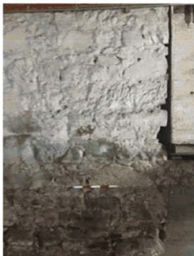
Figure 22: Roughly worked stone wall, 79 Collins Street.
