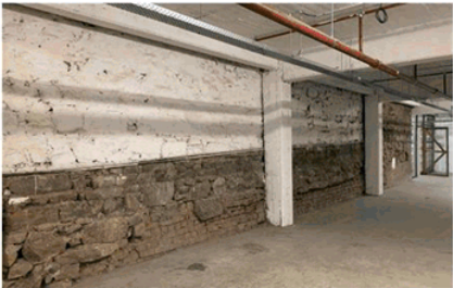
Figure 4 - Sandstone and brick walls to basement. (Source: Purcell)
