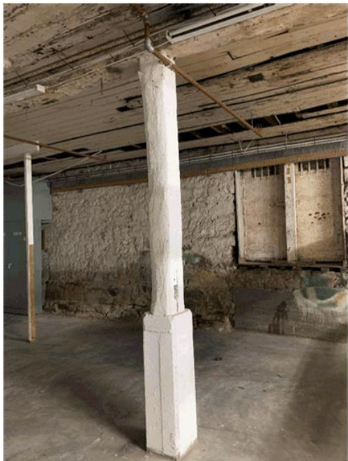
Figure 15 - Modified timber column to basement on concrete post. Concrete infill to exterior sandstone wall visible. (Source: Purcell)
