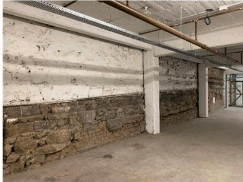
Figure 14 – Sandstone and brick dividing wall between 81 and 79 Collins Streets basements. (Source: Purcell)
