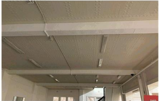
Figure 5 - Detail of pressed metal ceiling to ground floor. (Source: Purcell)
