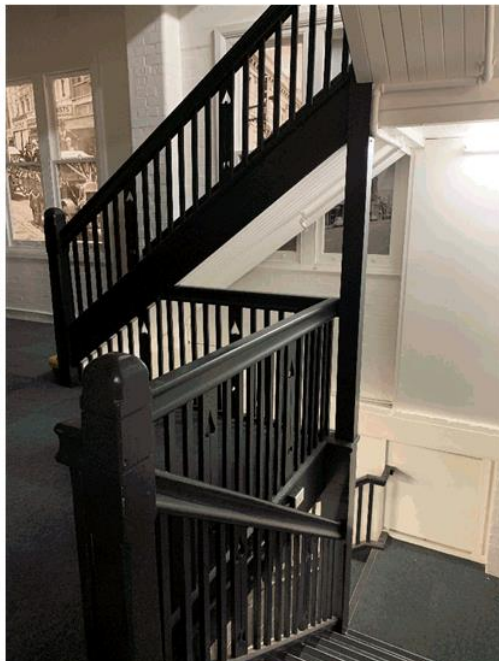
Figure 16 - Detail of timber balustrades on stair between Ground floor and Level 01. (Source: Purcell)
