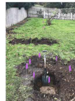
Reference image: Existing sewer I.O. and line location
