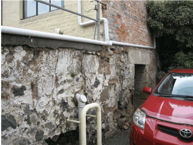
The c.1841 retaining wall and basement to the stables. Source: Council image
