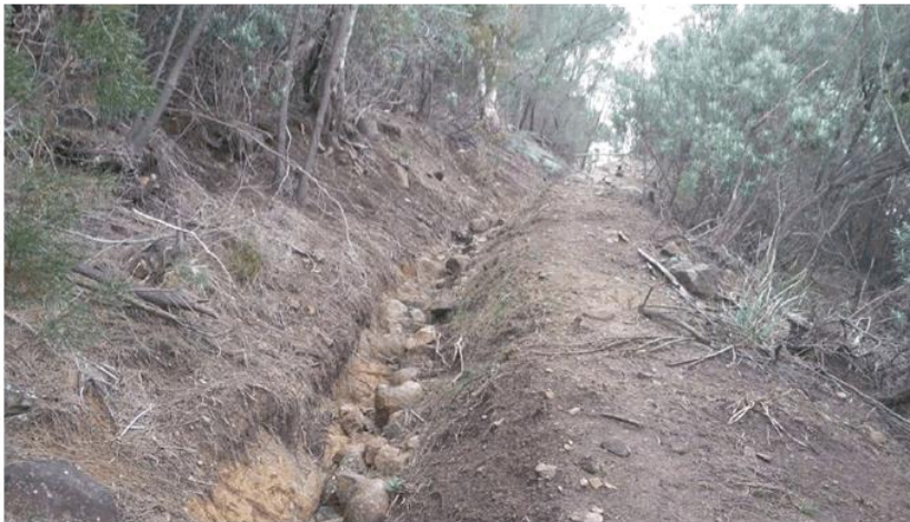
Image 3: Cut-off drain on 21B Enterprise Road
