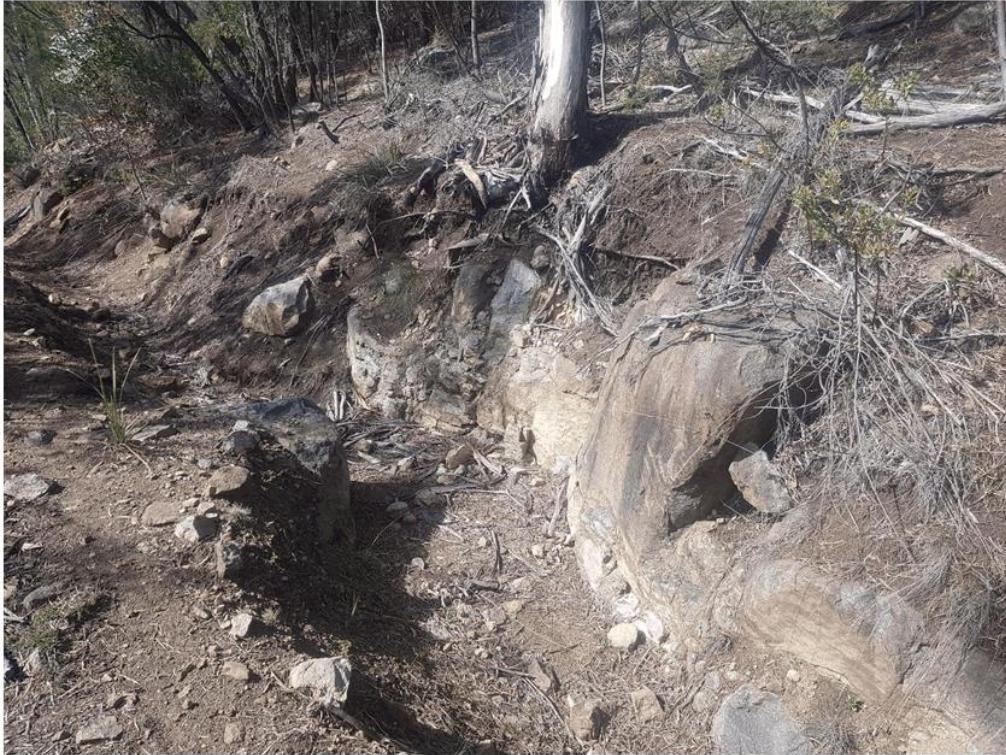
Figure 7: Bedrock exposed in cutoff drain at the base of the block
