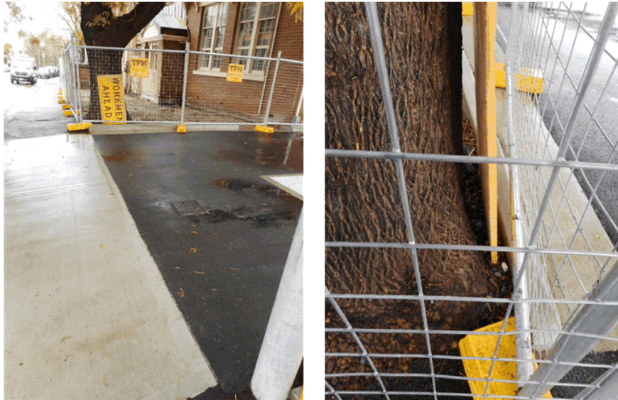
Figure 2. Recently completed hard surfaces immediately beside the ash trunk. Grate of a substantial stormwater infrastructure below the driveway is visible in the left image.
