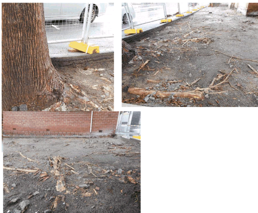
Figure 3. Large shallow roots (in excess of 100 mm in diameter) within the tree's structural root zone to the west and south have been broken and many others debarked reducing their functionality.
