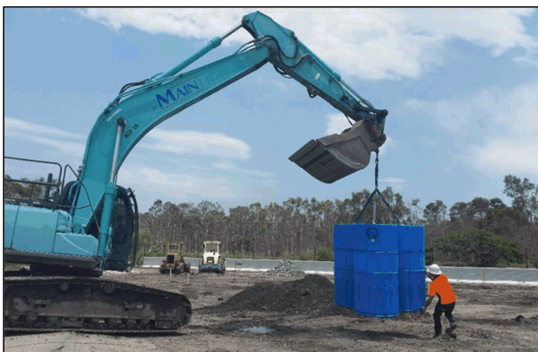
Figure 4.3: SPEL Hydrosystem (SHS.1000) installation using onsite digger
